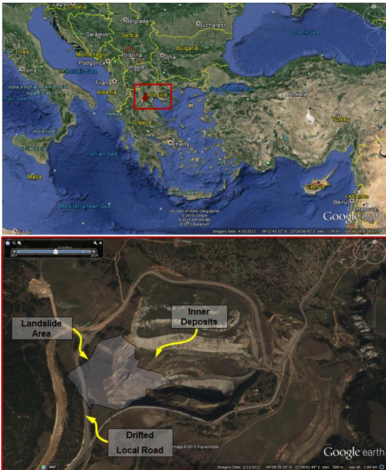
Figure 1. Position of landslide (up – red pin inside the red rectangle) and aerial photograph of the coal mine 2 weeks before the landslide (down). The area that was later occupied by the landslide is indicated with the transparent shape.
