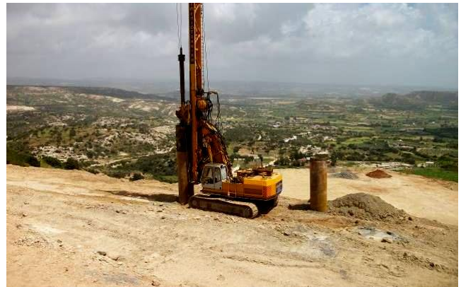
Figure 19. Installation of bored piles at the trimmed slope surface.
