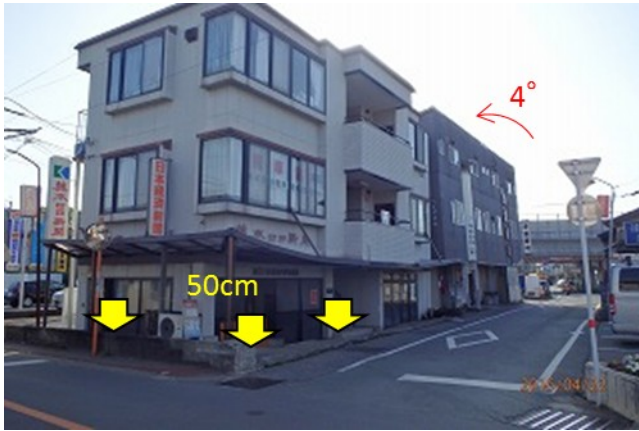
Figure 4. Liquefaction-induced damage to buildings in Karikusa district (Site 1 in Fig. 3) ( 32^{\circ} 45'35.70''N , 130^{\circ} 40'59.76''E ).
