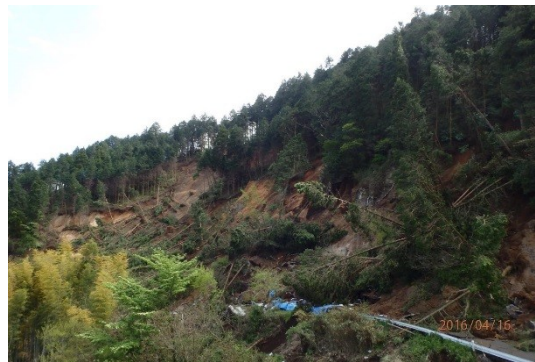
Figure 22. Slope failure along prefectural road No. 28 (site 14 in Fig. 12) ( 32^{\circ}50'32.96''N , 130^{\circ}55'40.65''E ).
