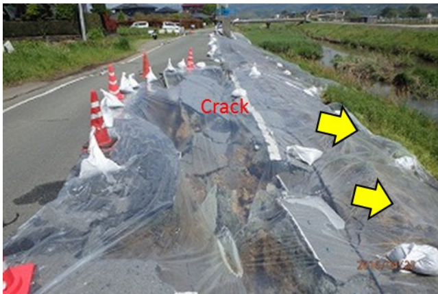
Figure 6. Liquefaction-induced damage to levee along Akitsukawa-River (Site 3 in Figs. 3 and 7) ( 32^{\circ} 46'43.56''N , 130^{\circ} 47'40.27''E ).
