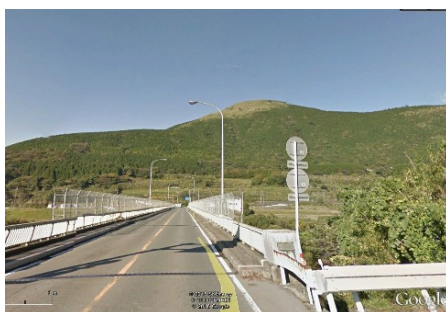
Before the failure (Google Earth)
