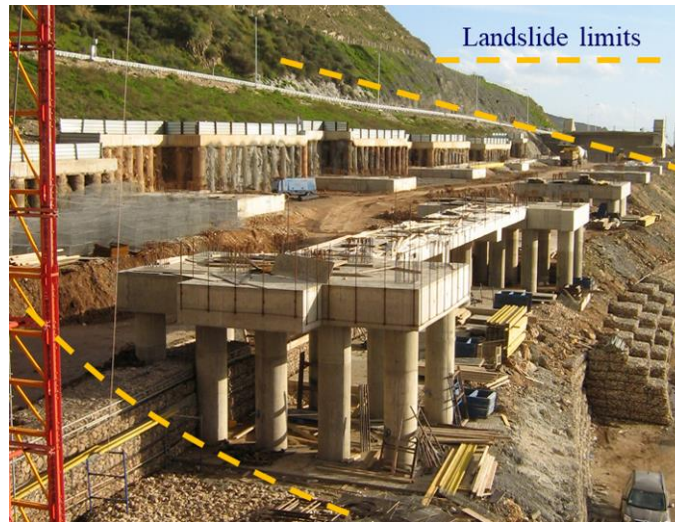
Figure 23. Assembling line of the right branch.
