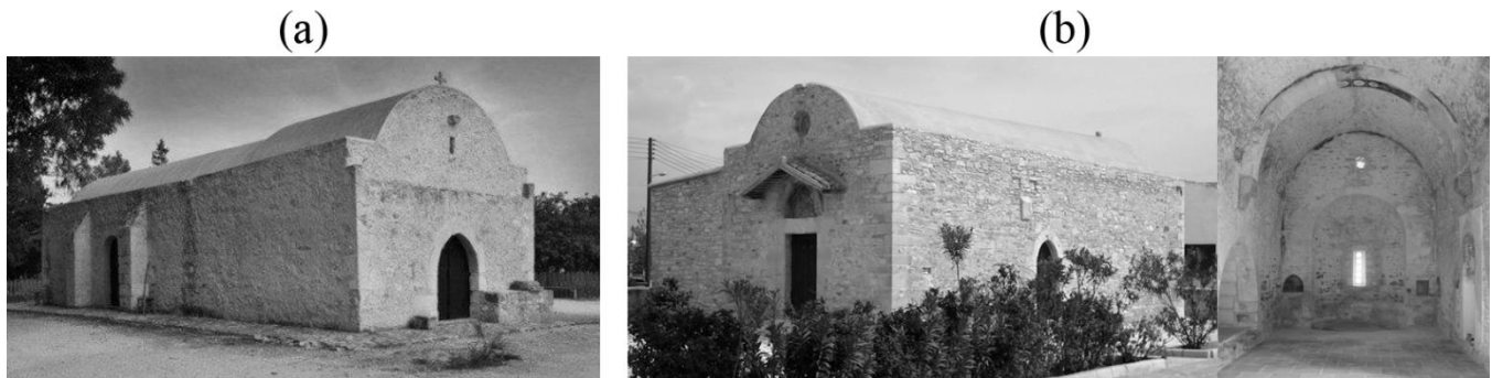
Figure 2. (a) Exterior view of the church of Agia Marina, Frenaros, Cyprus (15th century) and (b) exterior and interior view of the church of Saint Catherine, Larnaca, Cyprus (14th century).
