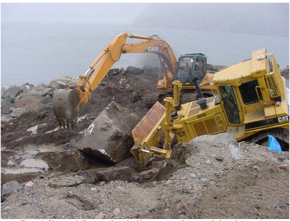
Figure 4. Photograph illustrating large boulders encountered at east end of trench excavation.
