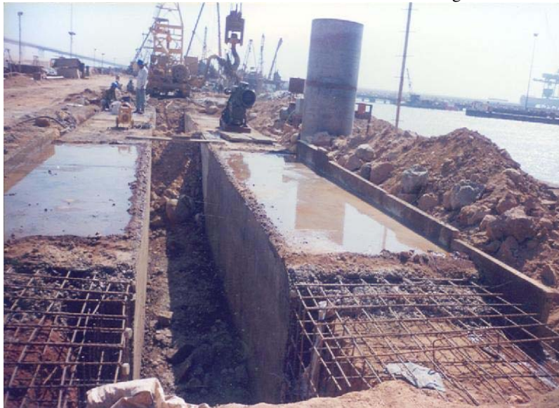
Figure 10. Construction Of Guide Walls For Diaphragm Wall.
