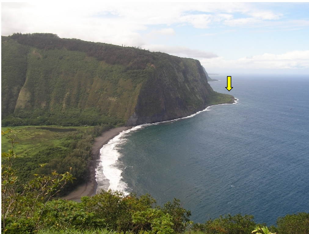
Figure 31. Location 8, Waipi'o Valley cliffs. Debris from an older slide (arrow) intrudes into the sea in the background. Scars in the closer, truncated spur are apparently not a result of the earthquakes since the water is not muddy.
