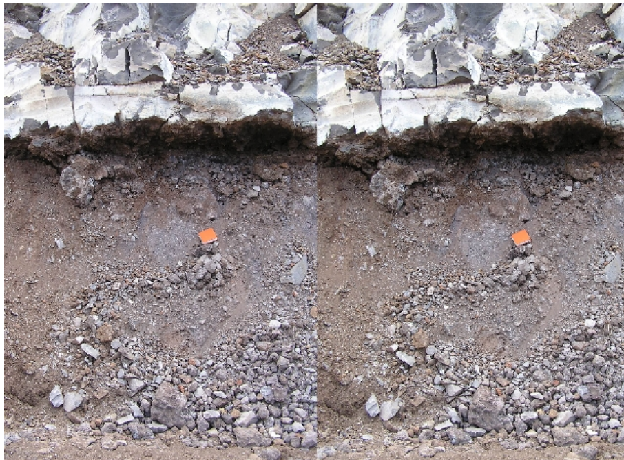
Figure 16. Location 25, Hwy 270 north of Kawaihae. 3-D stereo pair version of Figure 15. Cantilevered block of massive a'a basalt, undermined by clinker that raveled during the earthquakes.
