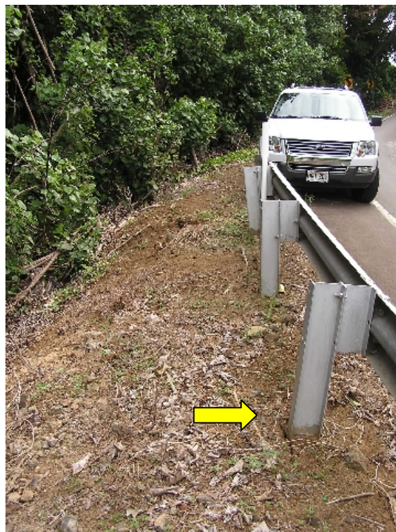
Figure 63. Location 18, Hwy 270 near Makapala, down slope side. Arrow indicates tension cracks and short head scarp 30 cm high at crest of steep and high fill slope.
