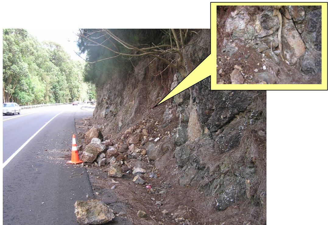
Figure 28. Location 9, Hwy 19 near Honoka'a. Weathered rock. Fractures occupied by tree roots, as shown in insert.
