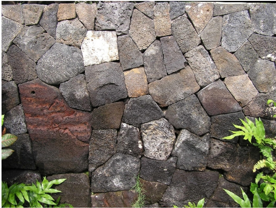
Figure 41. Location 33, Moku 'aikaua Church, Kailua-Kona. Finely constructed stacked rock perimeter wall.
