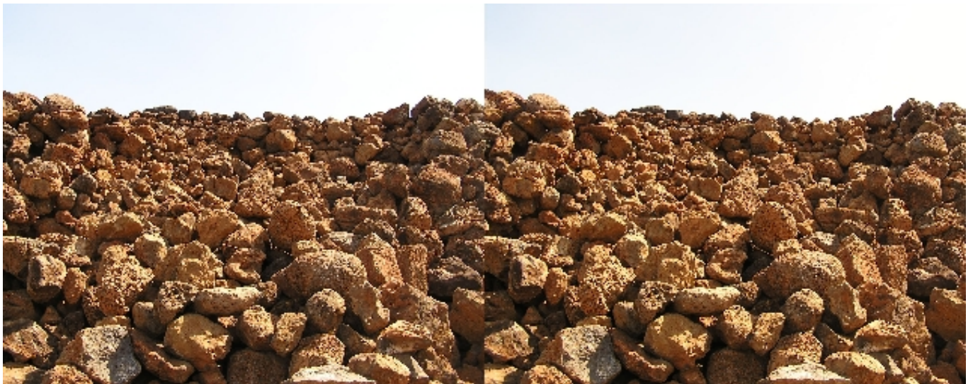
Figure 58. Location 29, slump failure in high rock wall of Pu'ukoholā heiau, west side. Stereo pair 3-D version of Figure 57.
