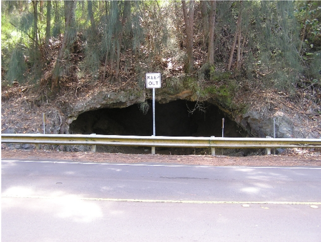
Figure 23. Location 7, Hwy 240, near Kapulena, north of Honokaa. Lava tube with apparently little rock fall from roof and walls.
