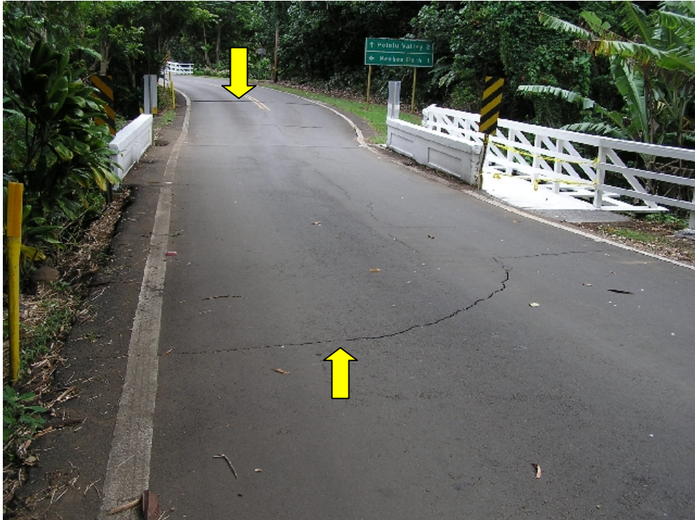
Figure 64. Location 20, bridge at approximately Mile Post 28, Hwy 270. Asphalt pavement cracked at approximately the cut/fill transitions of underlying subgrade.
