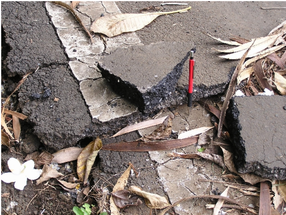
Figure 65. Location 20, bridge at approximately Mile Post 28, Hwy 270. Thrusting of asphalt concrete pavement.
