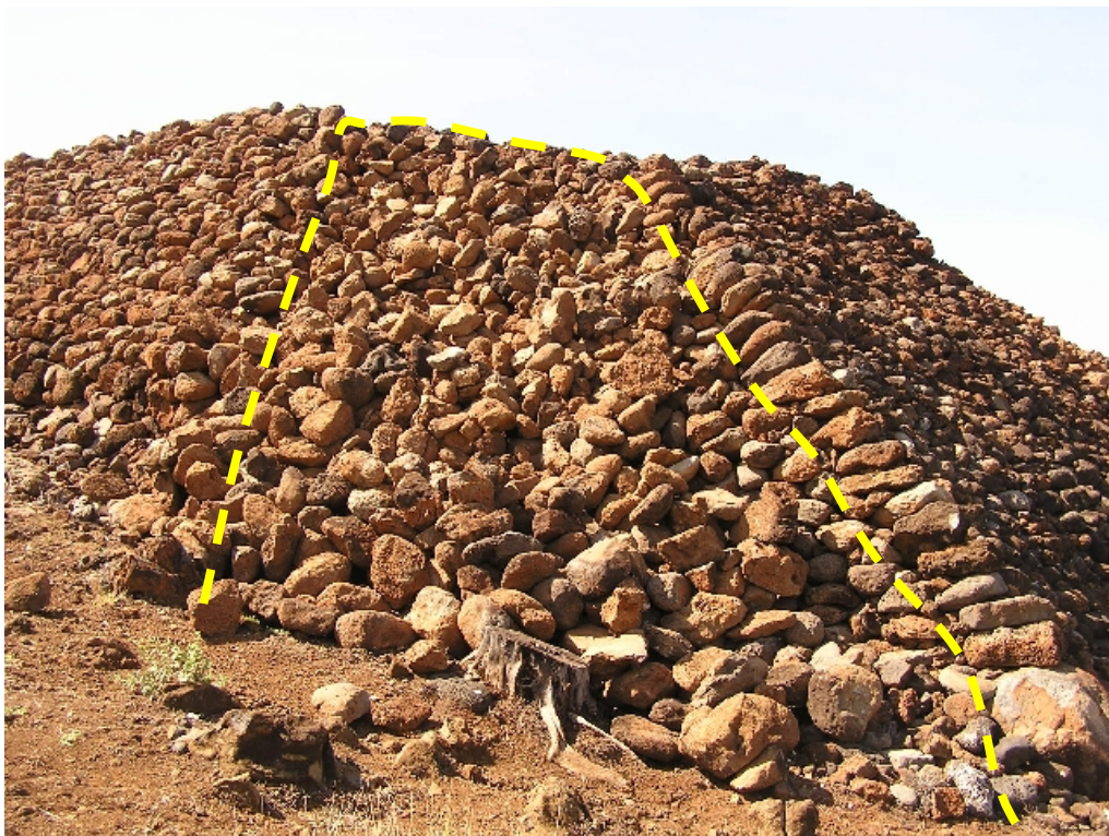
Figure 56. Location 29, Pu'ukoholā heiau, northeast corner. Dashed lines indicate boundary of ravel zone.
