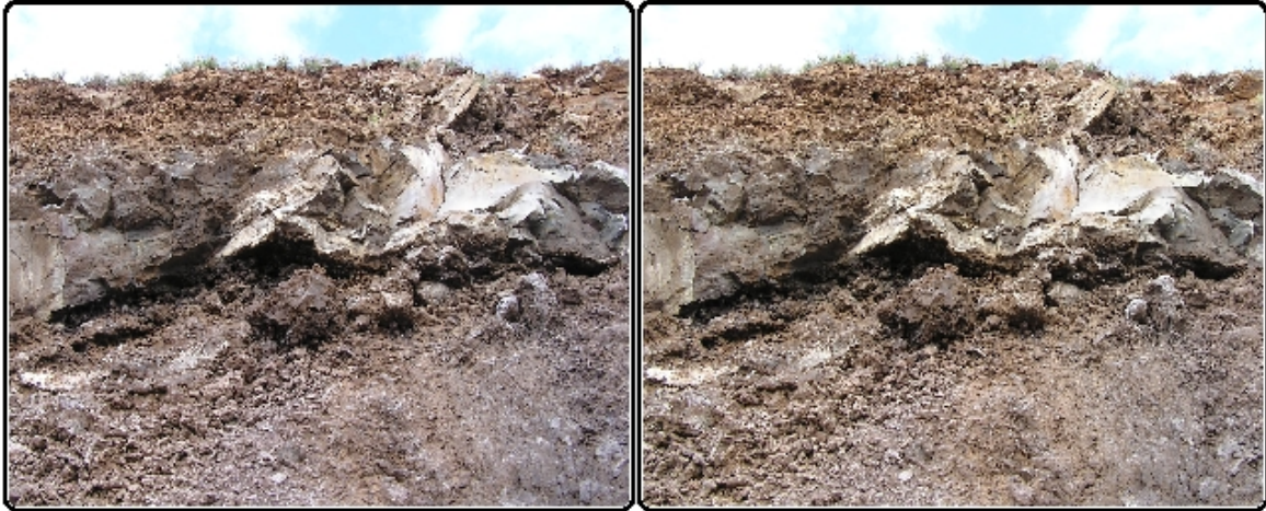
Figure 13. Location 25, near Kohala Ranch Estates, Hwy 270. 3-D stereo pair version of Figure 12. Road cut in mixed massive a'a and clinker.
