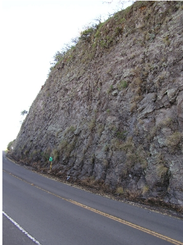
Figure 21. Location 13, Milepost 8, Hwy 250. Stable steep and high road cut.
