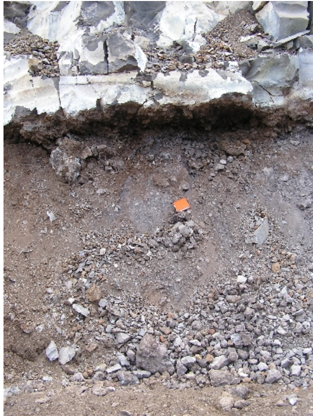
Figure 15. Location 25, Hwy 270 north of Kawaihae. Cantilevered block of massive a'a basalt, undermined by clinker that raveled during the earthquakes. See 3-D stereo images of Figure 16 and Figure 17.
