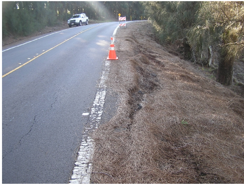
Figure 62. Location 15, north of Mile Post 9.4 Hwy 250. Slump failure of embankment on down slope side of road.
