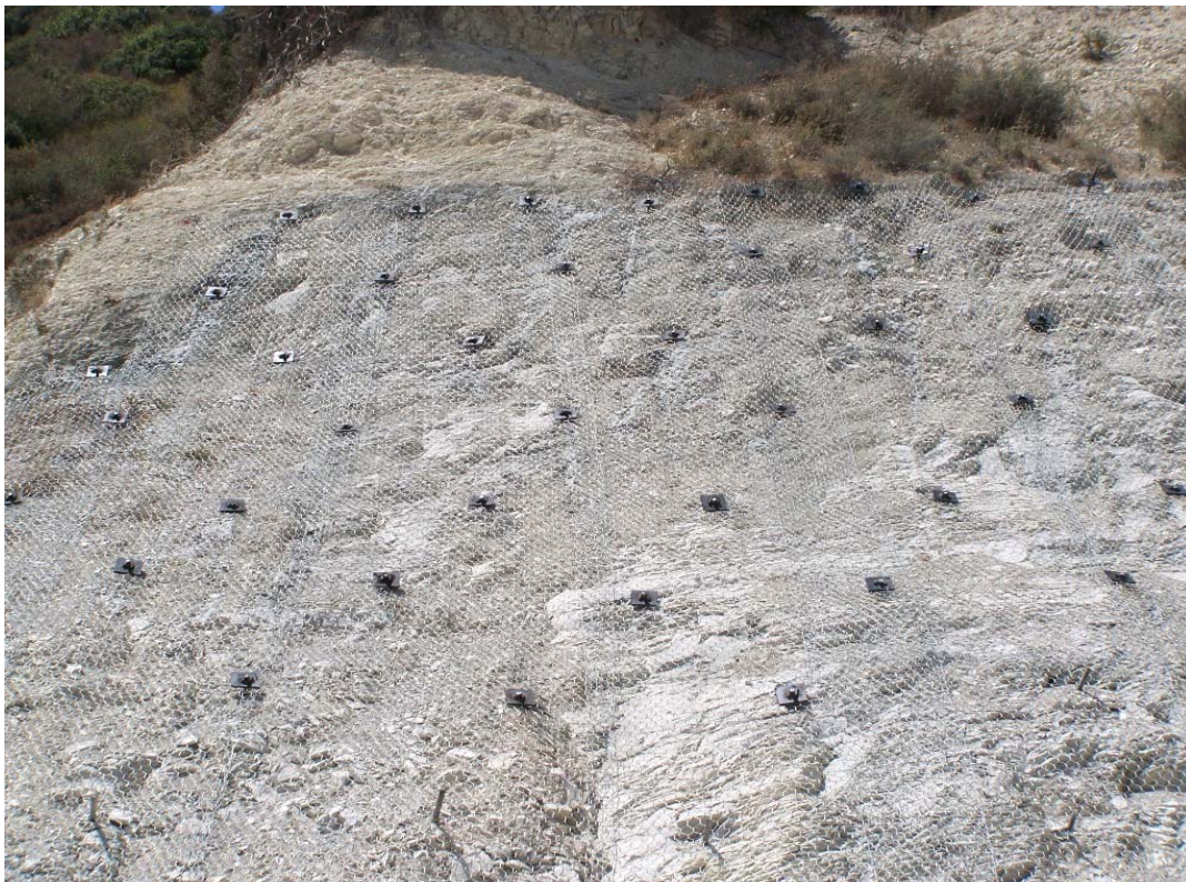
Figure 14. Completed Rock Bolts/nails and Wire Mesh Installation Along the Western Slope.
