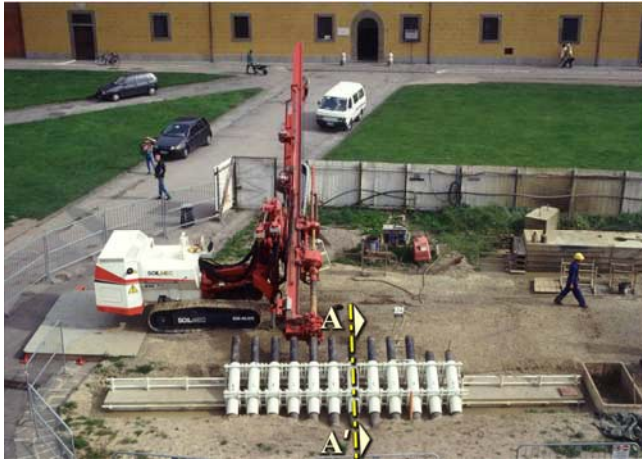
Figure 9. Holes for preliminary underexcavation.
