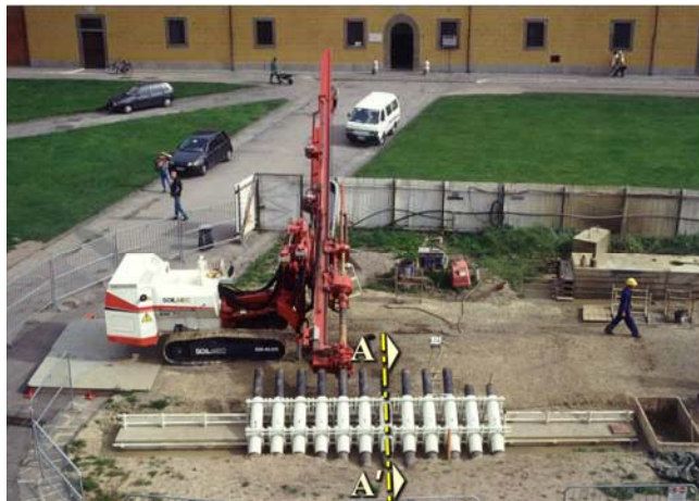
Figure 9. Holes for preliminary underexcavation.
