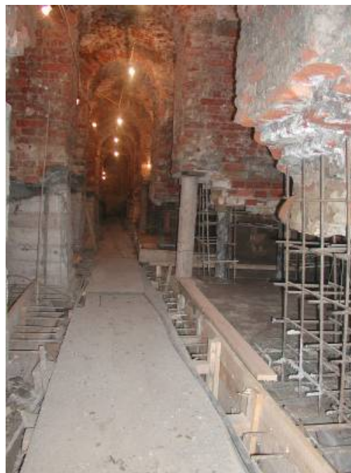
Figure 17. Deepening of the basements by 1.0-1.5 m.
