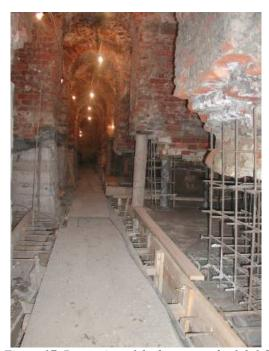
Figure 17. Deepening of the basements by 1.0-1.5 m.
