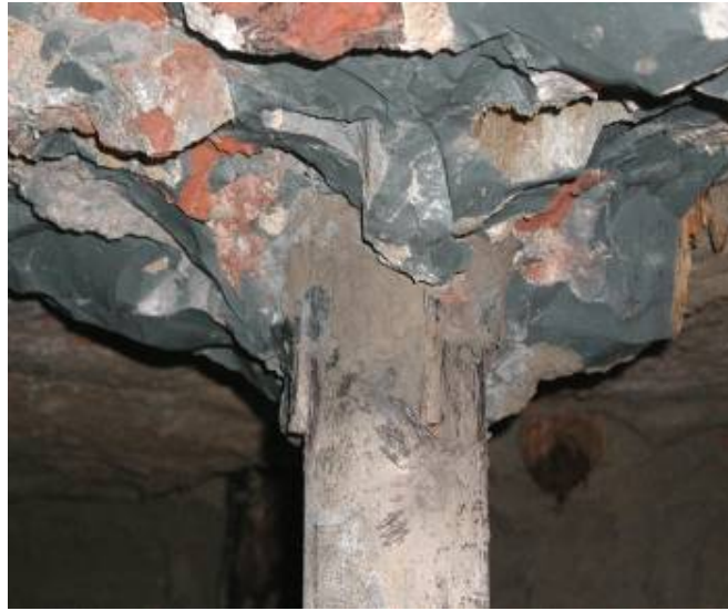
Figure 18. Bored pile with tube reinforcement viewed from underneath foundation.
