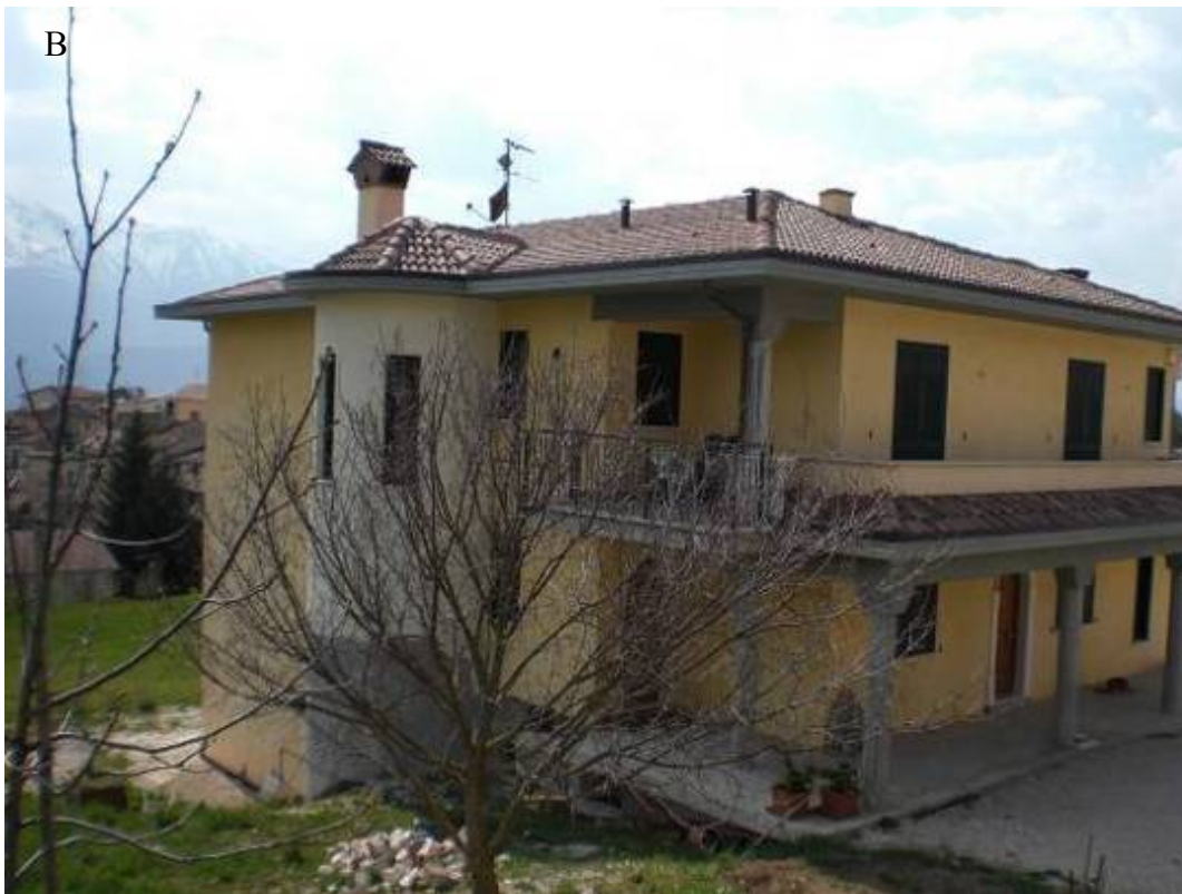
Figure 86. Poggio Picenze. (B) Undamaged RC house (D0) close to the (C) monumental church (D3).
