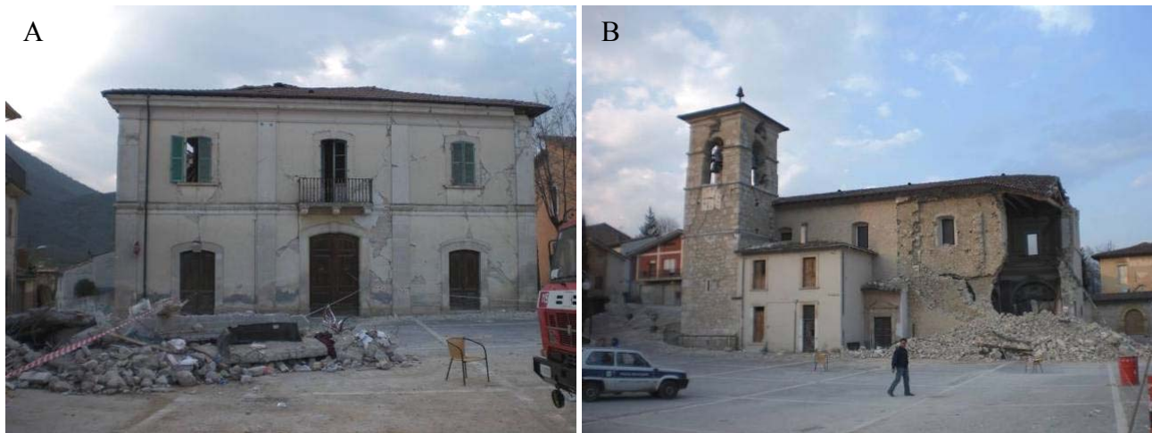
Figure 89. Villa S. Angelo, historic center with (A) masonry building crack,; (B) partly collapsed church.
