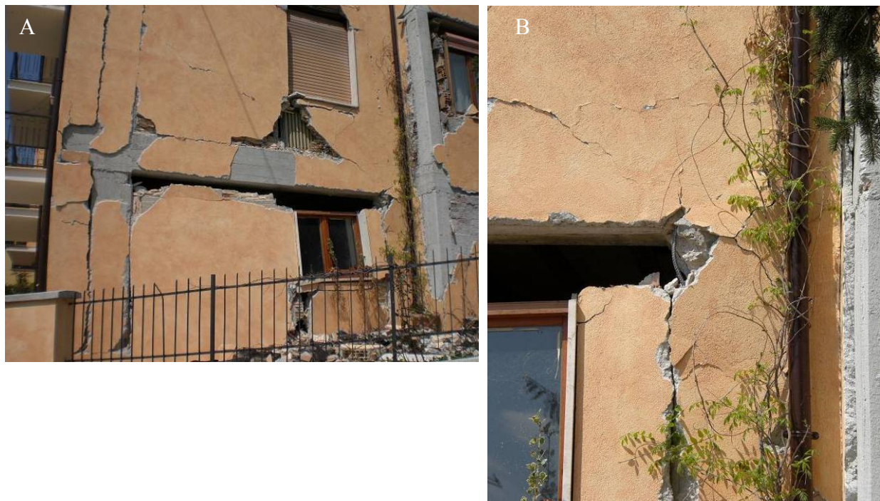
Figure 75. San Gregorio eastern part. (A) RC building with structural damage, (B) Detail of the damage to the beam-column connection.
