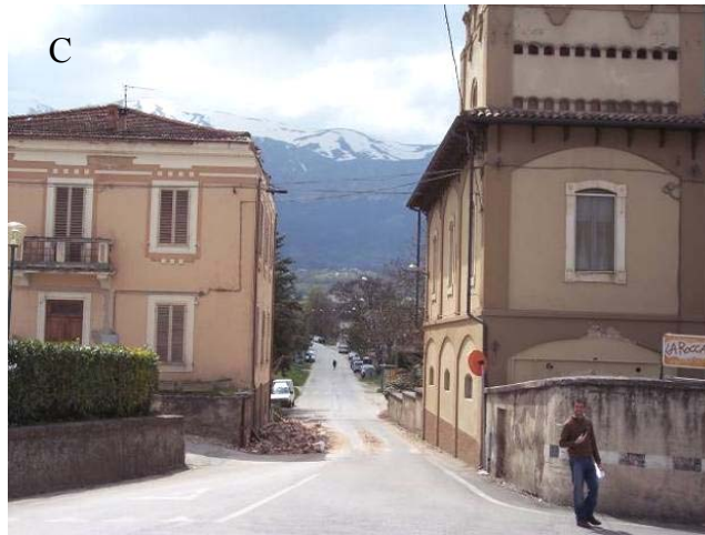
Figure 70. Monticchio. (C) D1 damage (fall of the cornice) on a masonry building.
