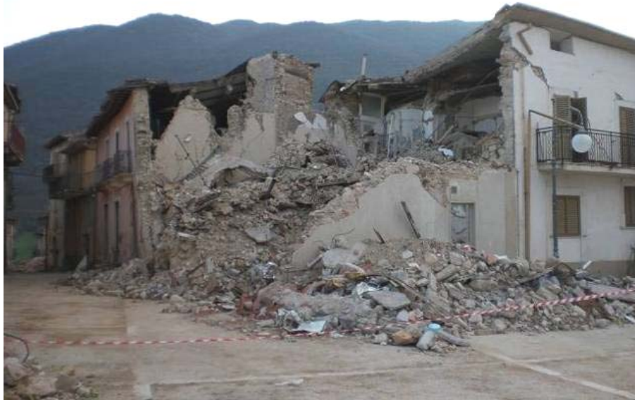
Figure 88. Villa S. Angel. (A) Collapsed masonry buildings (D5) in the historic center.
