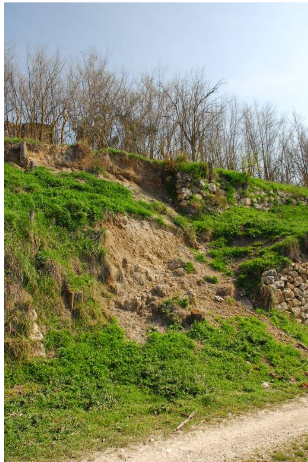
Figure 123. Shallow sloughing of regolith along road cut (southern flank of Castelnuovo N42.294, E13.628).
