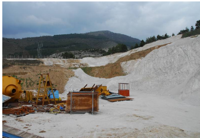
Figure 128. Quarry in Cataclasite with near vertical slopes segments up to approximately 15 m high, located northeast of Colle (42.435N, 13.330E).
