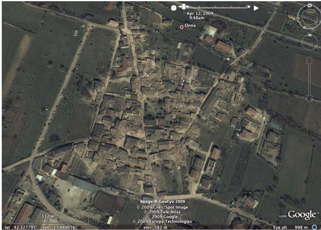
Figure 64. The village of Onna suffered D4–D5 damage in most of the unreinforced masonry structures. Reinforced concrete structures at the margins of the village performed well with only minor damage (D0-D2).
