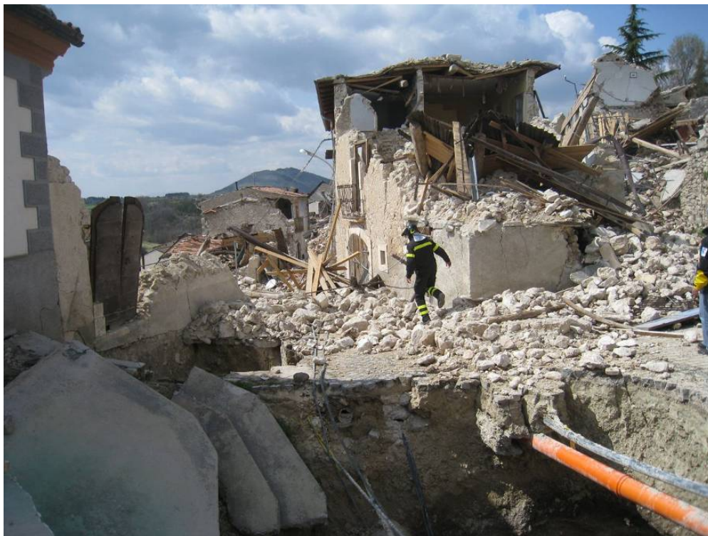
Figure 59. At the highest elevation of the hilltop town of Castelnuovo, almost all of the structures collapsed (D5) or were near collapse (D4). (42.2947°, 13.629°).
