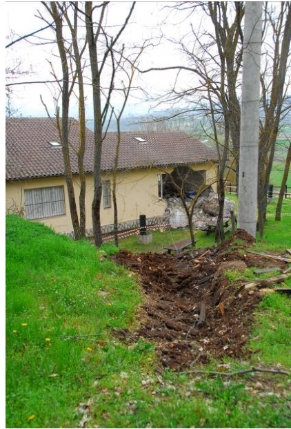
Figure 115. Last impact mark prior to impacting building at the Caves of Stiffe; the block trajectory was above the small tree (42.255N 13.547E).
