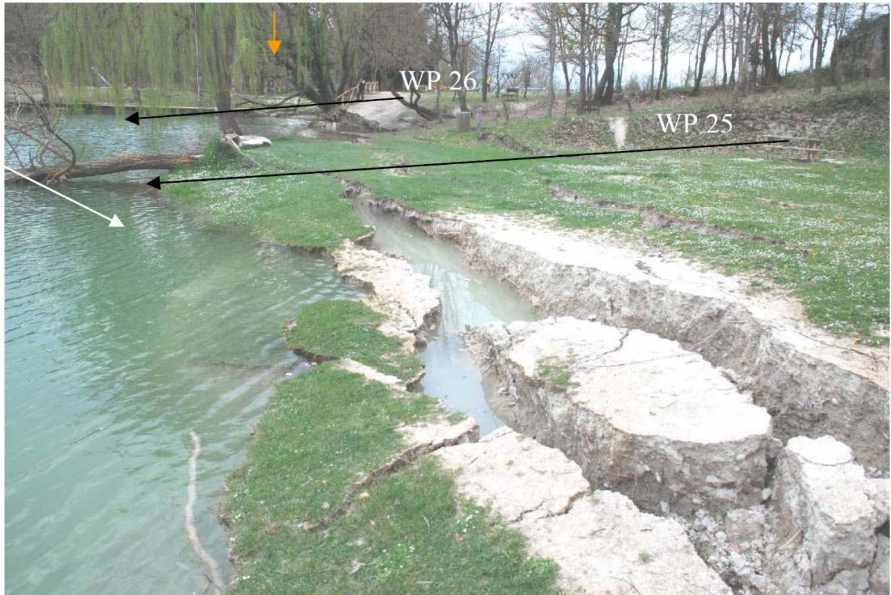
Figure 164. Blocks lying under the water (white arrow) were not included in the traverses (WP 25 and WP26). The orange arrow shows where the fence (and the slump below it) truncated the traverse at WP 27. (Photo E. Button).
