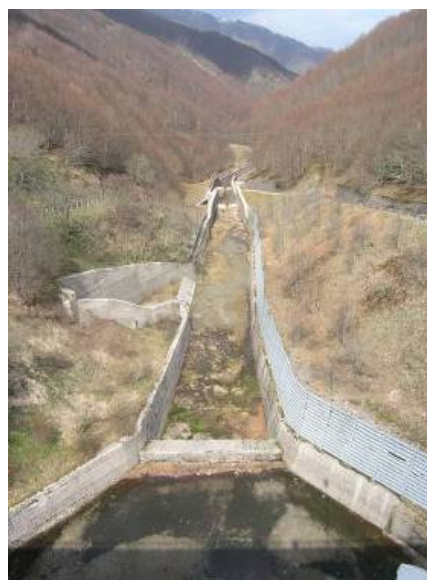
Figure 181. View of spillway of Rio Fucino dam (42.535047°N, 13.410323°E).
