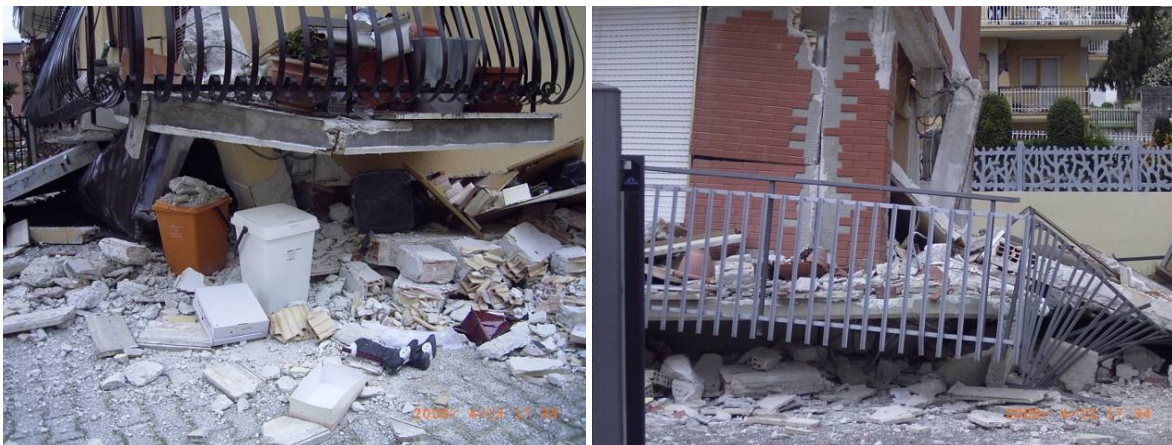
Figure 106. Example of D5 damage in the building at waypoints GB-27-1 and GB-28-1.
