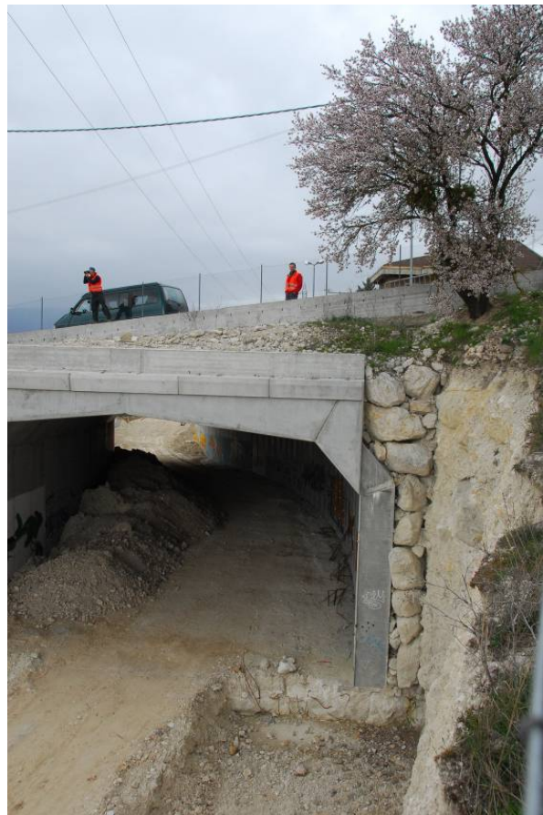
Figure 152. Boulder fill placed along side wall of cut-and-cover structure (42.358N 13.415E).
