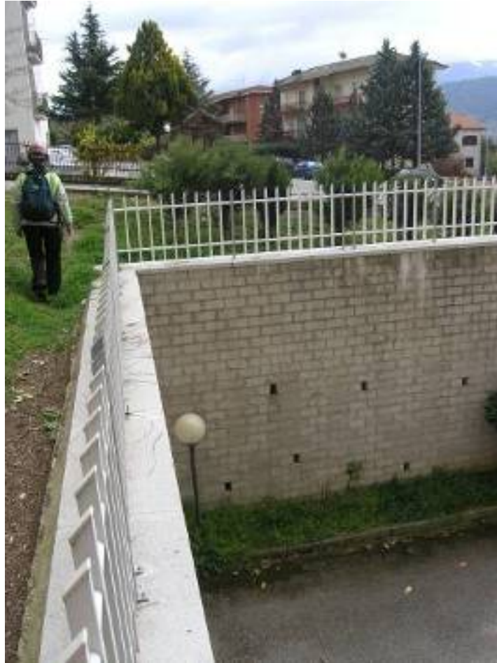
Figure 187. Undamaged wall at the severely shaken Pettino area (42.373050°N, 13.366106°E).
