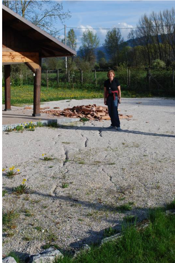
Figure 140. Ground fissures developed in alluvial floodplain directly south of central Onna and approximately 150 m from the Aterno River. Orientation of fissures is approximately parallel to the river (42.325N, 13.480E).
