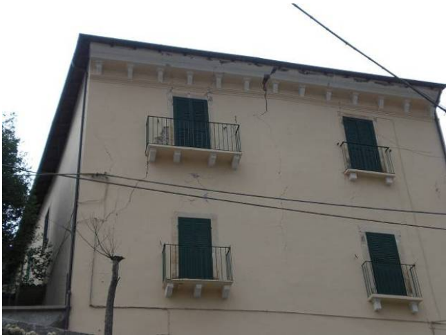
Figure 98. Goriano Sicoli. (A) Diagonal cracks in a masonry building (D3), (B) Partially collapsed masonry school (D4).
