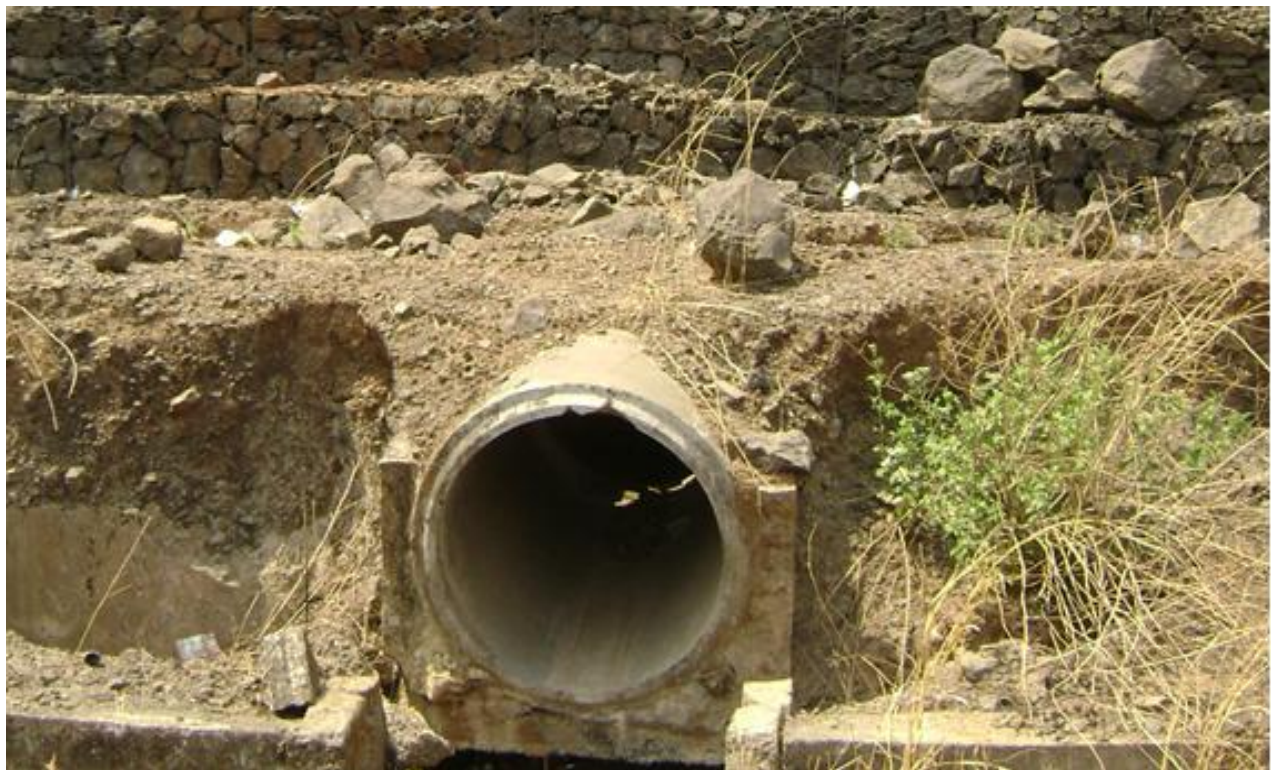
Figure 12. Pipe culvert without stepped chute.
