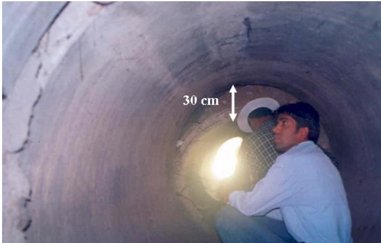
Figure 11. Dislodged pipe culvert.
