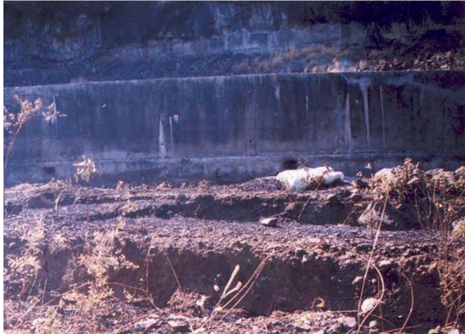
Figure 17. Subsidence of the embankment.
