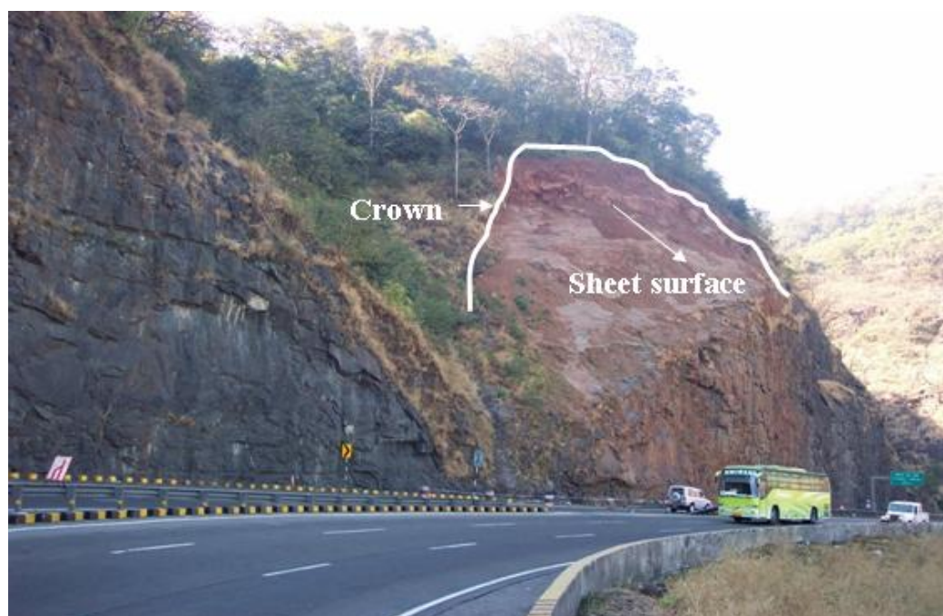
Figure 2. General view of rockfall and debris.
