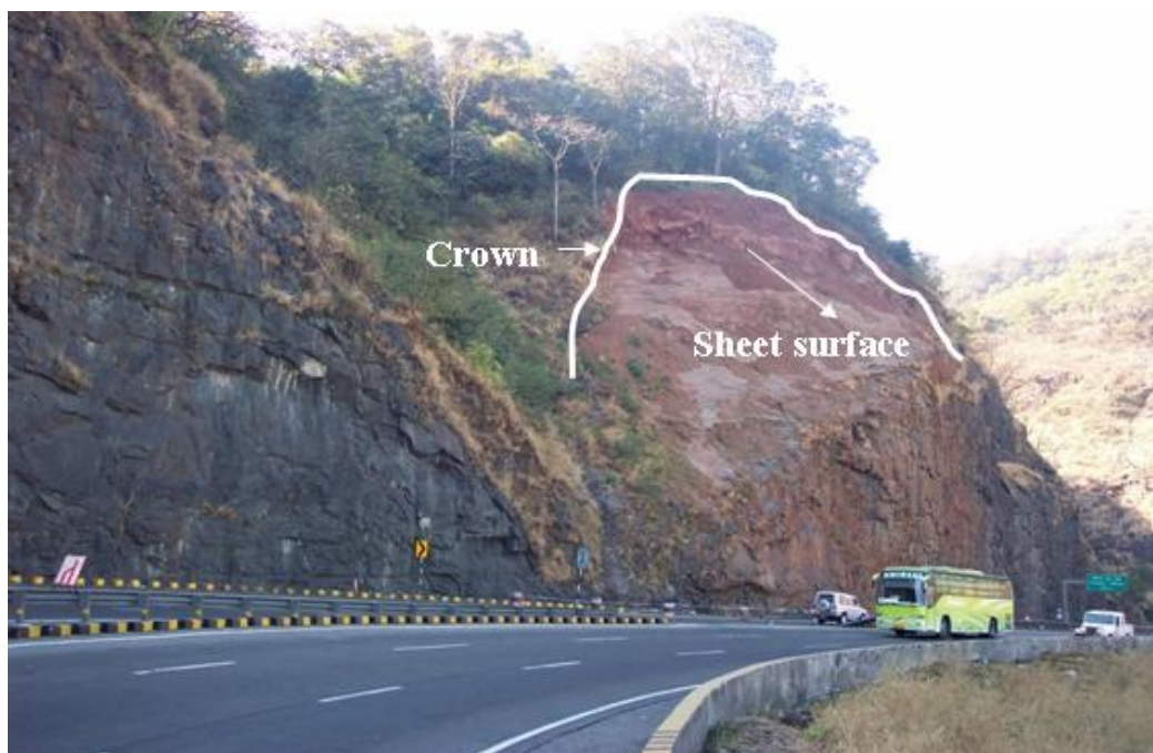
Figure 2. General view of rockfall and debris.
