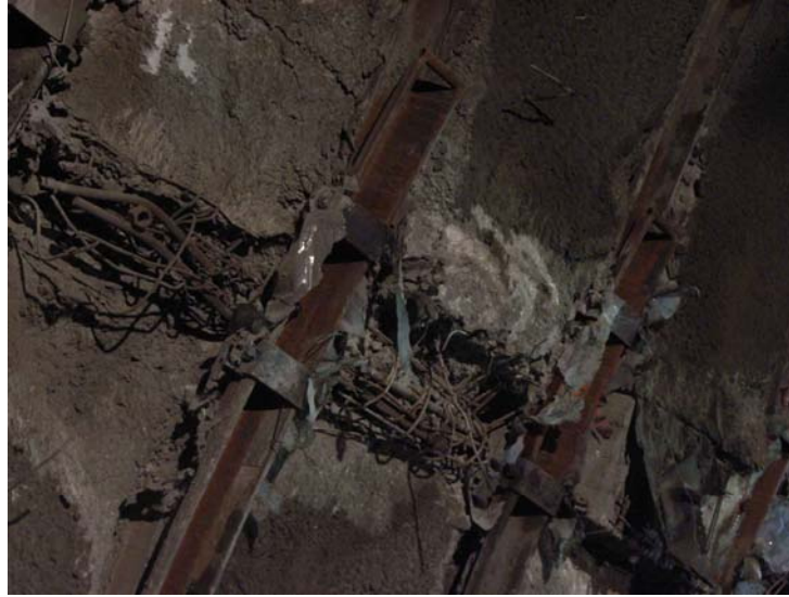
Figure 17. Detail of deformable element 6 at chainage 1443 m prior to casting of final lining.
