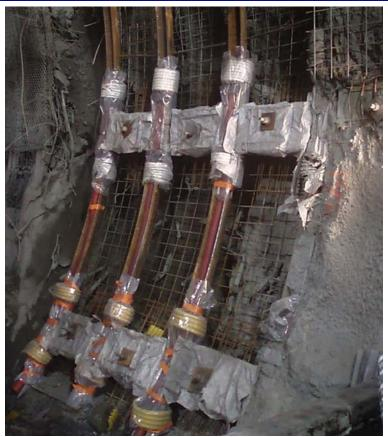
Figure 8. Detail of the installation of the TH steel sets and HiDCon elements.
