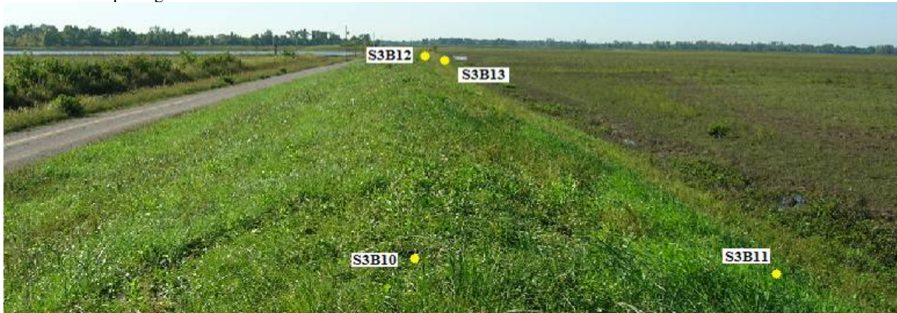
Figure 20. Brevator boring locations.
