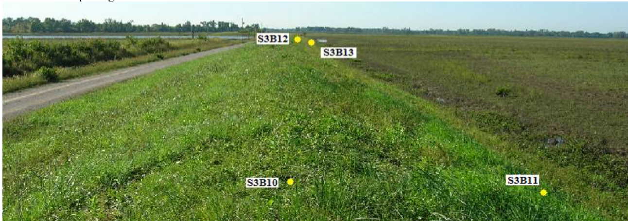
Figure 20. Brevator boring locations.
