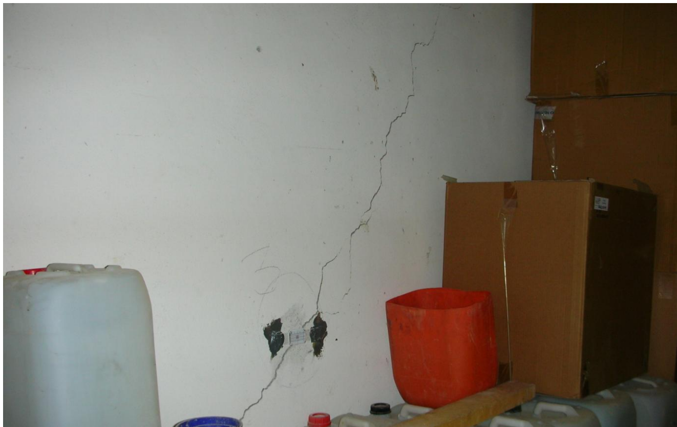
Figure 2. Wall damage inside the warehouse.
