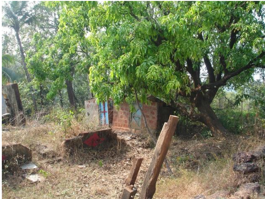
Figure 6. Tilted trees and cracked brick walls observed along the slope.
