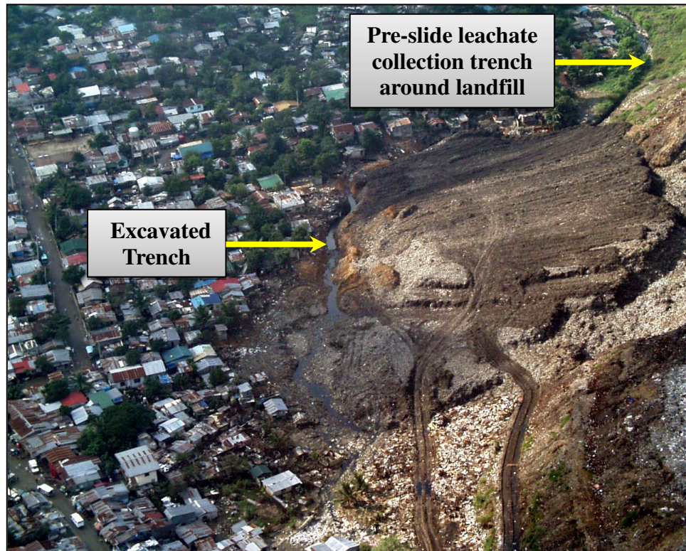
Figure 5. Slope failure showing new and existing leachate trenches along slope toe (photo by S.M. Merry).
