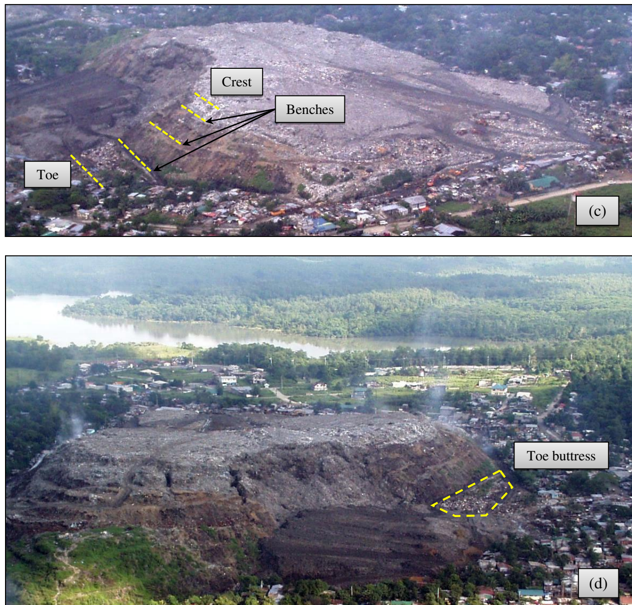
Figure 6. Slope geometry and failure surface after failure (a) evidence of seeping leachate, (b) representative slope inclination, (c) location of slope benches, (d) toe buttress (photos by S.M. Merry).
