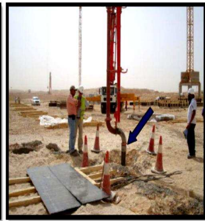
Figure 9.a. and b. Karst foundation bedrock treatments; cement grout injection, c. and d. high slump concrete filling.
