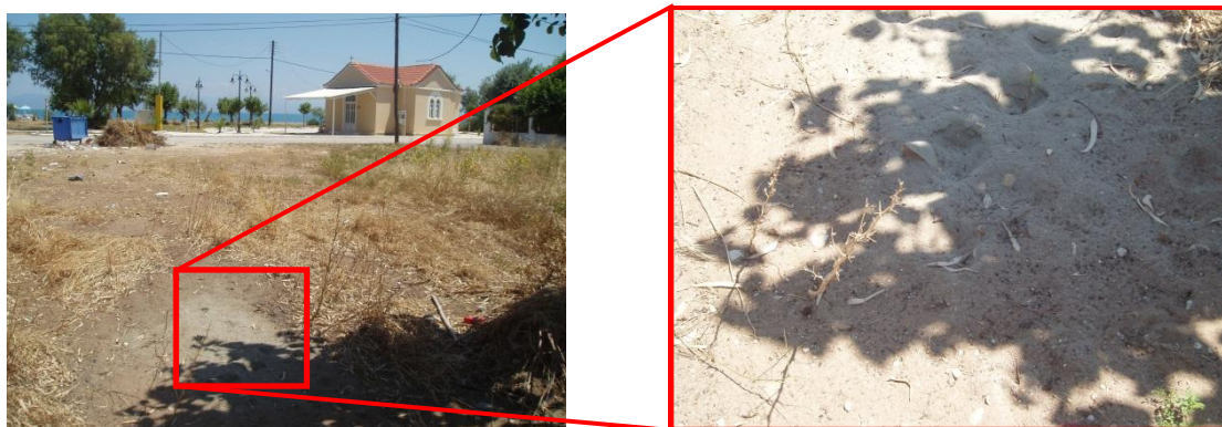
Figure 4. Marginal soil liquefaction at SITE-II, in the coastal zone of K. Achaia, following the 8-6-2008 earthquake. The ejected material is classified as gray silty sand (SM).
