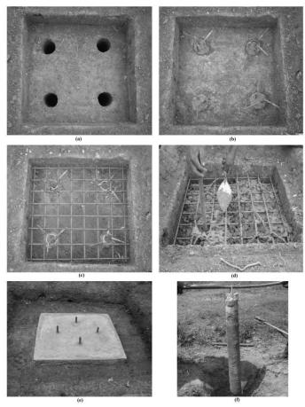
Figure 4. Stages of Construction Process of Pile Groups.
