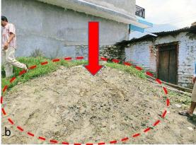
Figure 6. Typical effects of sinkhole formation on residential properties observed on June 2014 included the collapsed of (a) a cowshed and (b) a masonry kitchen.
