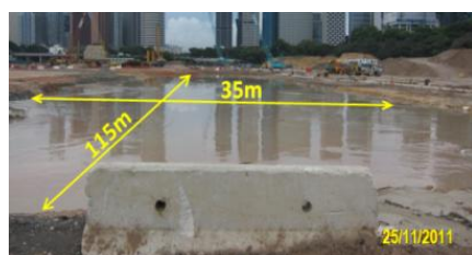
(b) Photograph of pond B (115 m x 35 m x 8 m) with slurry clay heaved from RL94 m to RL102 m.
