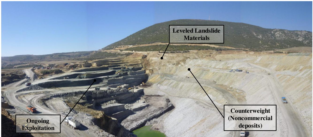
Figure 13. Aspect of the coal mine area after completion of counterweight construction and leveling works (March 2012).
