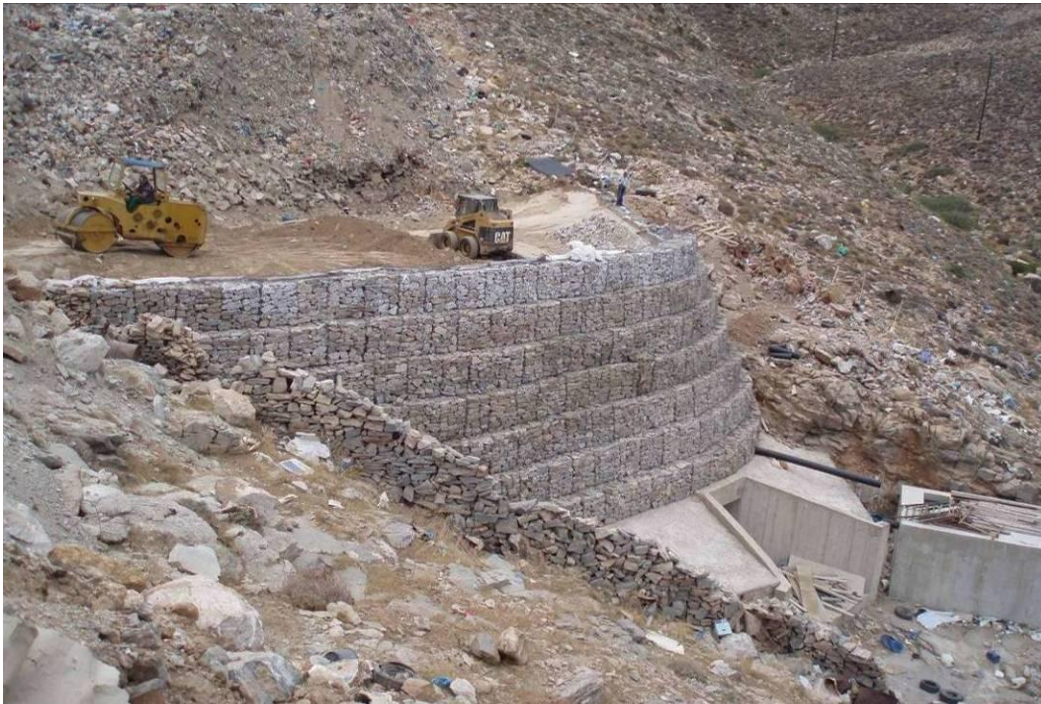
Figure 12. Construction of reinforced earth during landfill final closure.
