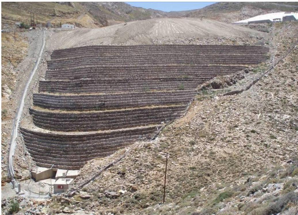
*Figure 13. View of Syros uncontrolled landfill after final closure.*
