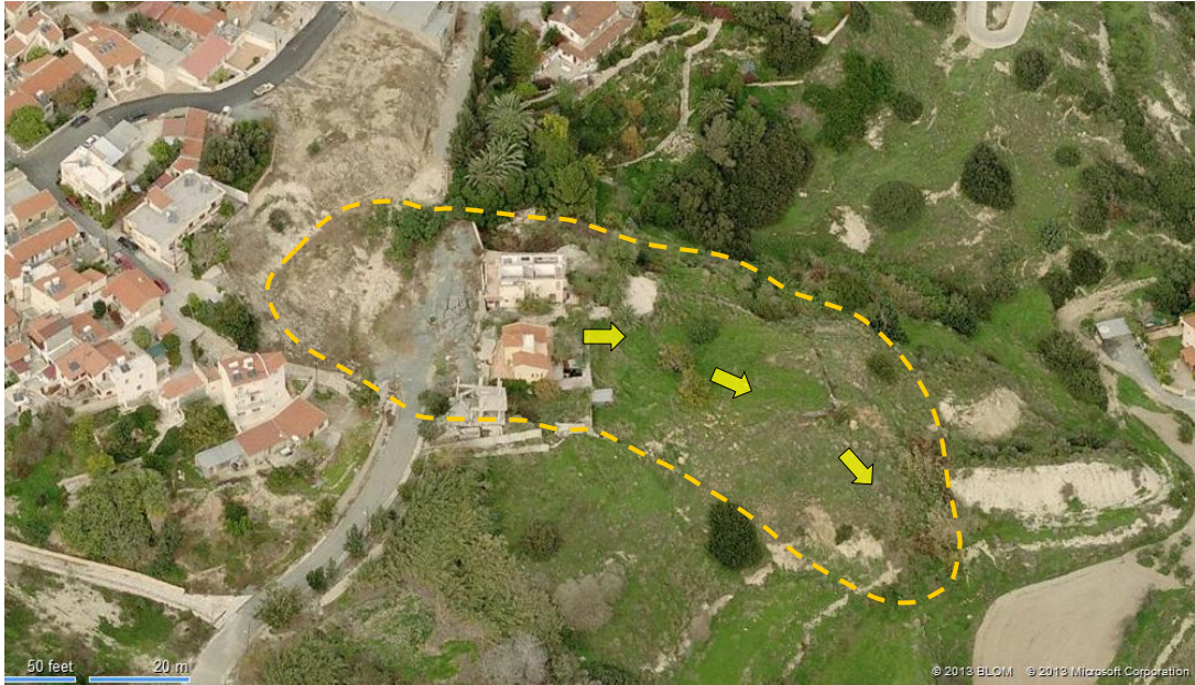
Figure 1. Aerial view of the Pissouri landslide. Dashed line indicates the border of the sliding mass. Notice the distorted road and the damaged residential buildings resting on the sliding mass.
