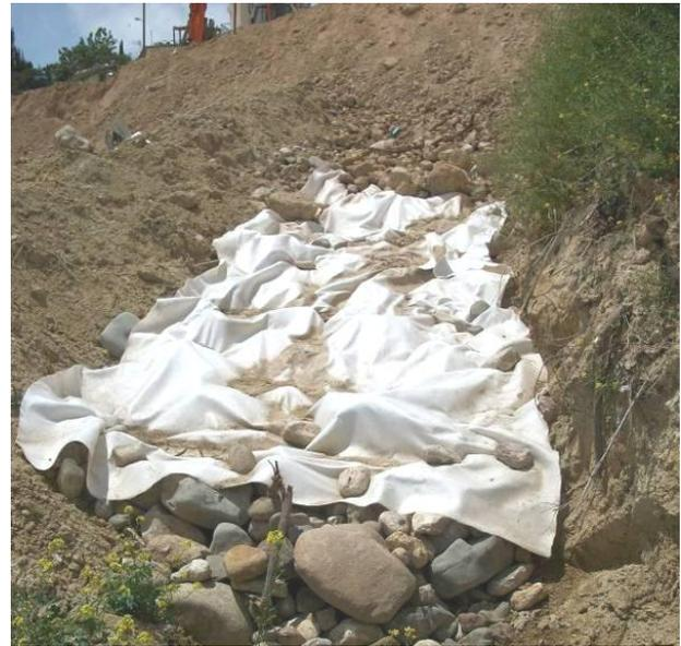
Figure 21. Trench drains filled with cobles wrapped in geotextile filter collect and dispose the groundwater.
