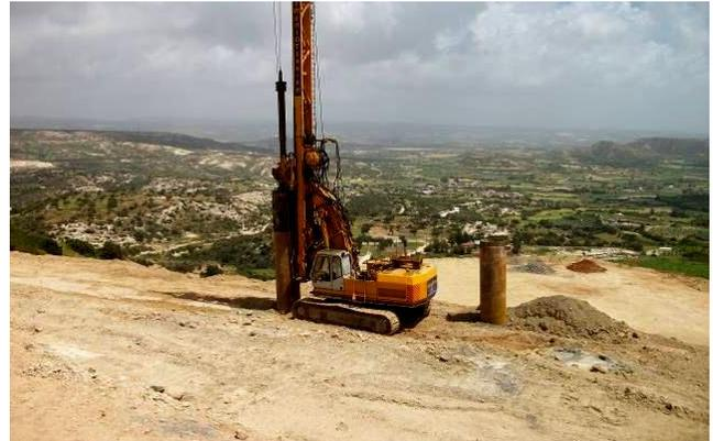
*Figure 19. Installation of bored piles at the trimmed slope surface.*
