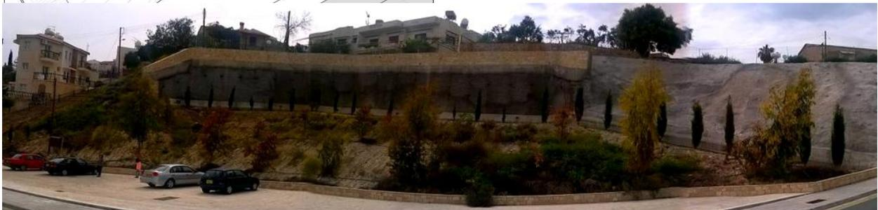
Figure 22. The landslide back scarp area after its stabilization by installing a permanent anchored wall.
