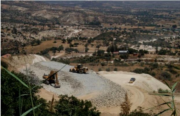
*Figure 18. Construction of the Buttress fill*
