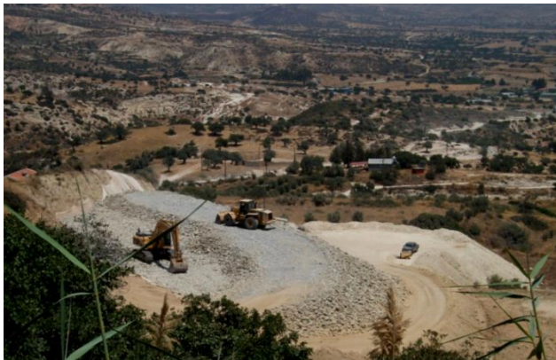
Figure 18. Construction of the Buttress fill
