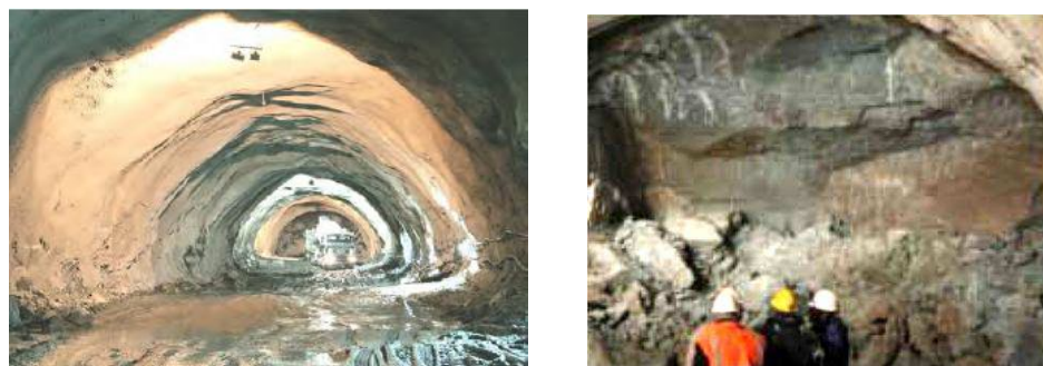
Figure 16. Response of molassic rocks during tunnelling of the “Egnatia odos” tunnels. Left: Structurally controlled overexcavation - Ag.Paraskevi tunnel (after Dounias et al 2010). Right: structurally controlled instability at tunnel face in thick sandstone layers separated by sparse thin siltstone intercalations (after Marinos et al. 2013)
