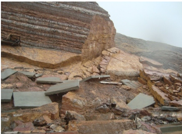
Figure 4. Top photo provides an overall view of the slope face prior to sliding and the extent of two episodes of sliding on June 4 th and October 11 th 2010. The lower frames, except the lower right corner view, show sliding during Cyclone Phet, while the lower right corner view shows the resulting slope face after the final collapse on October 11 th 2010. The sliding along the bedding and a vertical joint, a free release plane along the overspilled wadi, is an obvious reason of sliding during cyclone Phet.
