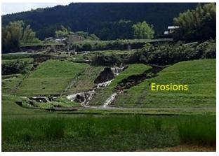
Figure 21. Damage to road embankment along prefectural road No. 28 (site 13 in Fig. 12) (32°50'36.63"N, 130°55'24.48"E).
