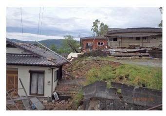
Figure 16. Ground displacement-induced damage to a residential house (Site 8 in Fig. 12) (32° 47'24.96"N, 130° 49'12.75"E).
