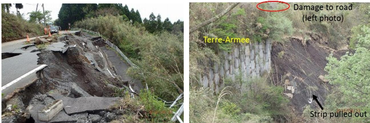
Figure 35. Damage to road embankment and reinforced retaining wall (Terre-Armee) (site 22 in Fig. 26) ( $32^{\circ} 52'52.01''N$ ,  $131^{\circ} 00'14.84''E$ ).
