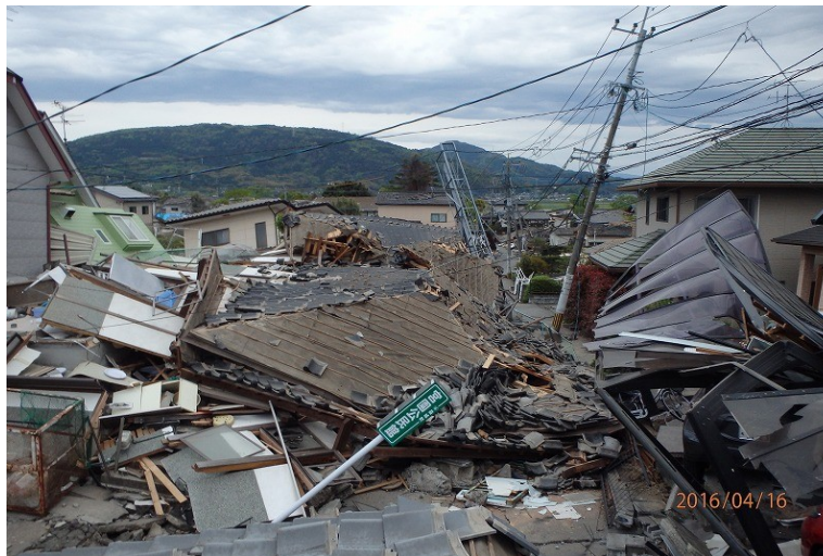
Figure 13. Damage to residential houses in Mashiki Town (Site 7 in Fig. 12) ( 32^{\circ} 47'16.38''N , 130^{\circ} 48'58.47''E ).
