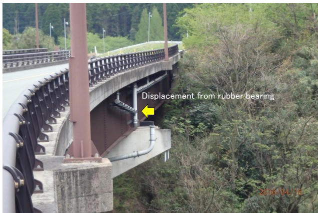
Figure 24. The girder of Ohkiri-hata Bridge moved about 1-1.5m (Site 14 in Fig. 12) ( 32^{\circ} 50'32.63''N , 130^{\circ} 55'43.10''E ).
