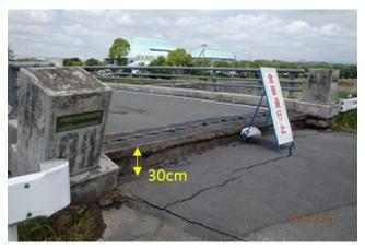
Figure 8. A large gap at bridge girder due to settlement of embankment (Site 4 in Fig. 3) (32° 47'2.15"N, 130° 49'17.70"E).
