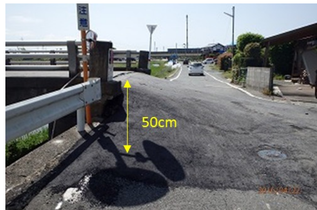
Figure 9. Temporary restoration work (filled slope) for settlement of levee (Site 5 in Figs. 3 and 7) ( 32^{\circ}46'44.47''\text{N} , 130^{\circ}47'45.43''\text{E} ).
