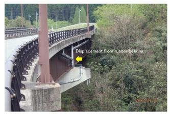
Figure 24. The girder of Ohkirihata Bridge moved about 1-1.5m (Site 14 in Fig. 12) (32°50'32.63"N, 130°55'43.10"E).
