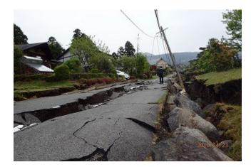
Figure 32. Damage to the road in residential area developed by filling (Site 21 in Fig. 26) (32° 52'43.89"N, 130° 59'58.89"E).
