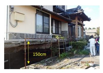
Figure 36. Ground depression-induced damage to the residential house (Site 23 in Fig. 26) (32° 57'23.84"N, 131° 2'12.31"E).
