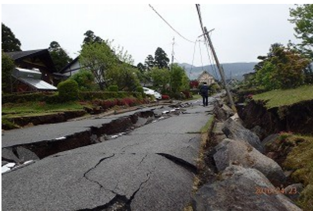
Figure 32. Damage to the road in residential area developed by filling (Site 21 in Fig. 26) ( 32^{\circ} 52'43.89''N , 130^{\circ} 59'58.89''E ).
