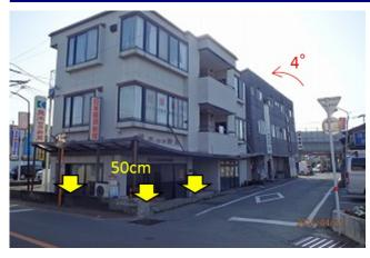
Figure 4. Liquefaction-induced damage to buildings in Karikusa district (Site 1 in Fig. 3) (32° 45'35.70"N, 130° 40'59.76"E).
