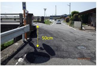
Figure 9. Temporary restoration work (filled slope) for settlement of levee (Site 5 in Figs. 3 and 7) (32° 46'44.47"N, 130° 47'45.43"E).
