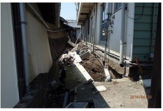
Figure 17. Ground displacement-induced damage to a residential house (Site 9 in Fig. 12) (32° 47'14.48"N, 130° 48'41.06"E).
