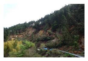
Figure 22. Slope failure along prefectural road No. 28 (site 14 in Fig. 12) (32°50'32.96"N, 130°55'40.65"E).
