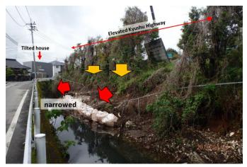
Figure 10. Damage to Kyushu Highway embankment (Site 6 in Figs. 3 and 7)  $(32^{\circ} 46'46.80"N, 130^{\circ} 47'39.40"E)$ .
