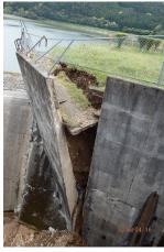
Figure 20. Damage to retaining wall and spillway retaining wall (site 12 in Fig. 12) (32°50'29.22"N, 130°55'55.83"E).
