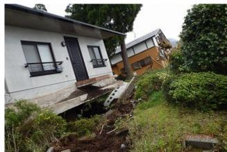
Figure 33. Damage to the house in residential area developed by filling (Site 21 in Fig. 26) (32°52'45.06"N, 131°00'1.44"E).
