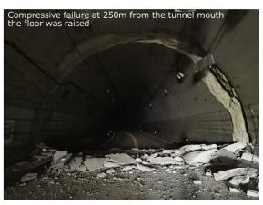
Figure 25. Tawarayama tunnel suffered from axial compression failure (Site 16 in Fig. 12) (32°51'35.68"N, 130°58'6.86"E).
