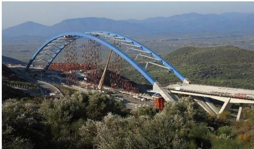
Figure 14. Removal of the temporary towers.
