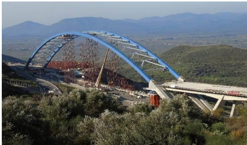
Figure 14. Removal of the temporary towers.
