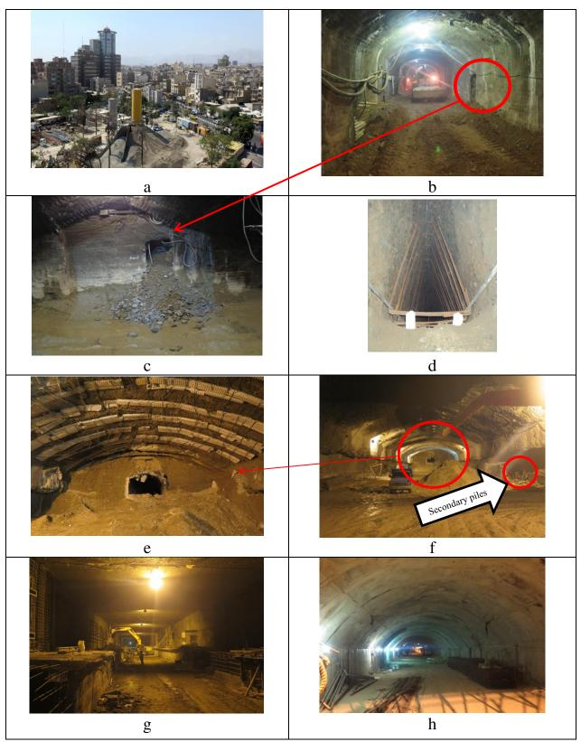
Figure 5. Actual stages of the station construction.
