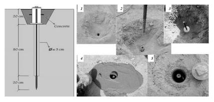
Figure 8. Installation of monitoring equipment 1-Making a ditch on the ground surface(depth of about 20 cm), 2- locating the pod in ground (depth 80 cm), 3- setting the pin in the pod,4- covering near the pin head by concrete, 5- positioning the protective cap on it).
