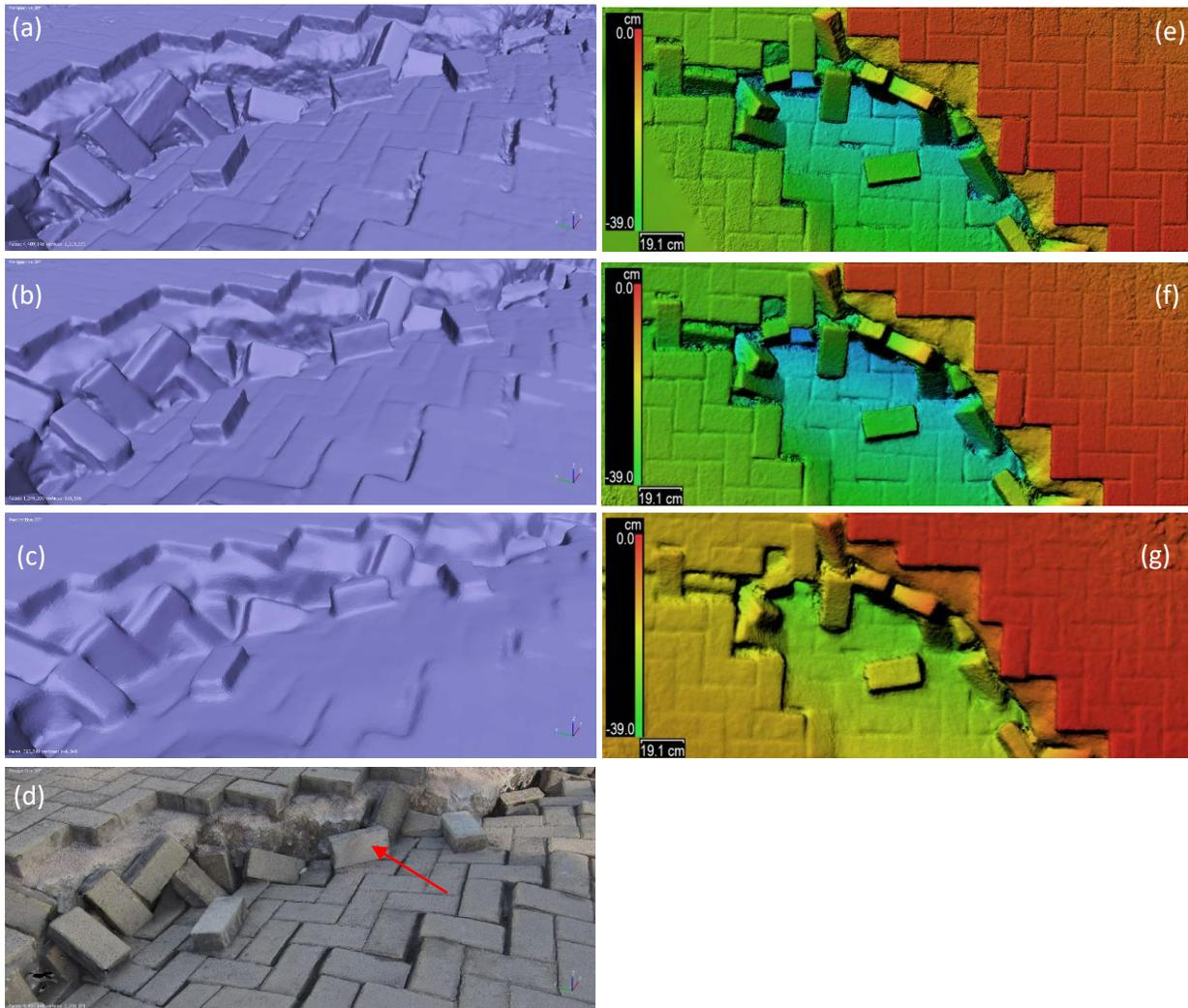
Figure 8. 3D model of cracked pavement with bricks at the Vasiliki port of Lefkada due to lateral movement of the seafront at a resolution of (a) 1.13 mm/pix (point density: 77.7 points/cm<sup>2</sup>); (b) 2.27 mm/pix (point density: 19.4 points/cm<sup>2</sup>); (c) 4.54 mm/pix (point density: 4.86 points/cm<sup>2</sup>). (d) photorealistic model of (a). Plan view at a resolution of (e) 1.13 mm/pix; (f) 2.27 mm/pix; (g) 4.54 mm/pix. Arrow points to brick being discussed in main text.
