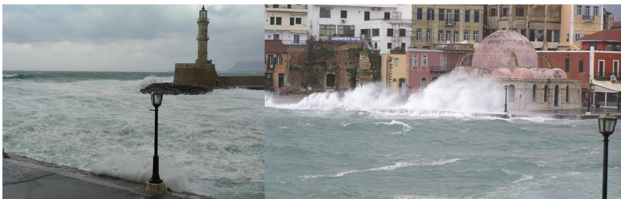
Figure 4. The wave disturbances inside the old Venetian harbour during a winter storm in 2011. Photos provided by the Natural Disasters and Coastal Engineering Laboratory (NDCEL), TU-Crete, Greece.
