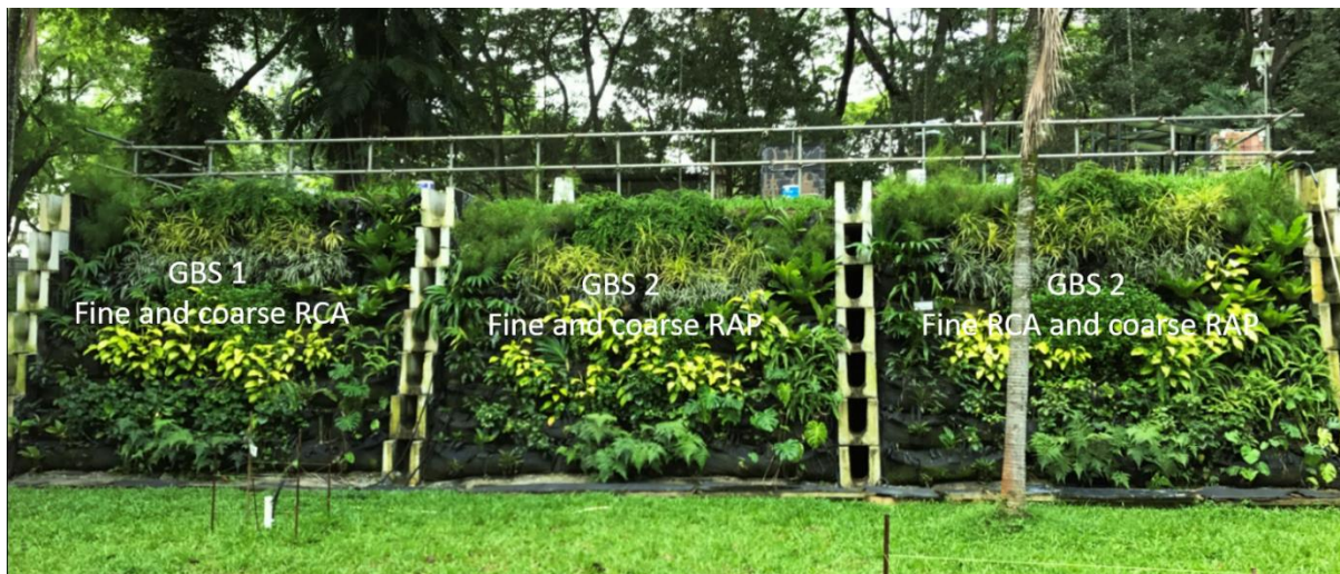
Figure 4. GBS at Orchard Boulevard.
