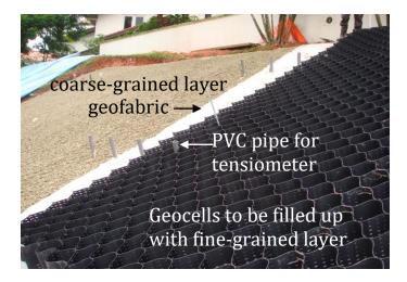
Figure 5. Laying of separator layer and fine-grained layer.
