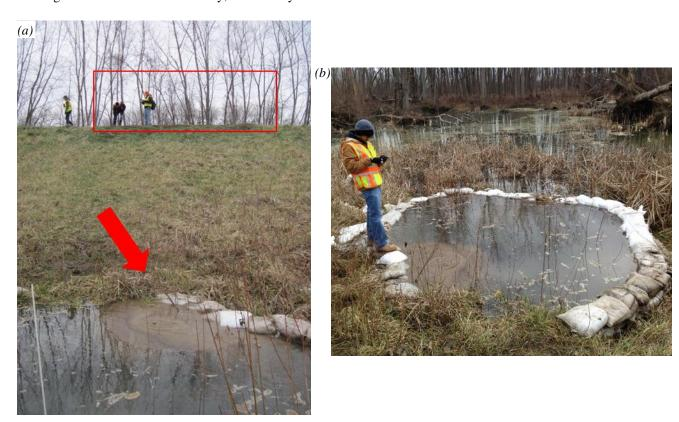
Figure 5. December 2015 flood reconaissance: (a) settlement of crown with active sand boil at toe of levee, (b) active sand boil with sand bag ring (Rutherford et al. 2016).
