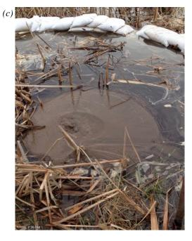
Figure 4. Observed damage during December 2015 flood event: (a) crown of levee, (b) 0.33 m diameter active sand boil, (c) active sand boil (Rutherford et al. 2016).
