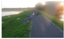
Figure 6. Photo series over time (upper left: 08.06.2013-10:37, initial break at the edge of the slope, upper right: 08.06.2013–14:10, horizontal shifts, bulge of the toe, lower left: 08.06.2013–20:51 continuing failure, lower right, 08.06.2013–20:55, continuing failure with the visual predictors (Grubert, 2013). Riverside of the levee is on the right for all photos.
