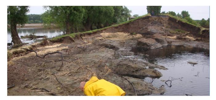
Figure 7. Photo of the cross-section of the breached levee (Grubert, 2013).
