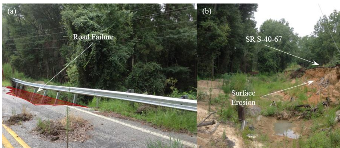
Figure 7. Failure of Dam A: (a) road failure of State Road S-40-67 (southeast view from S-40-67), and (b) surface erosion due to overtopping (west view from downstream).
