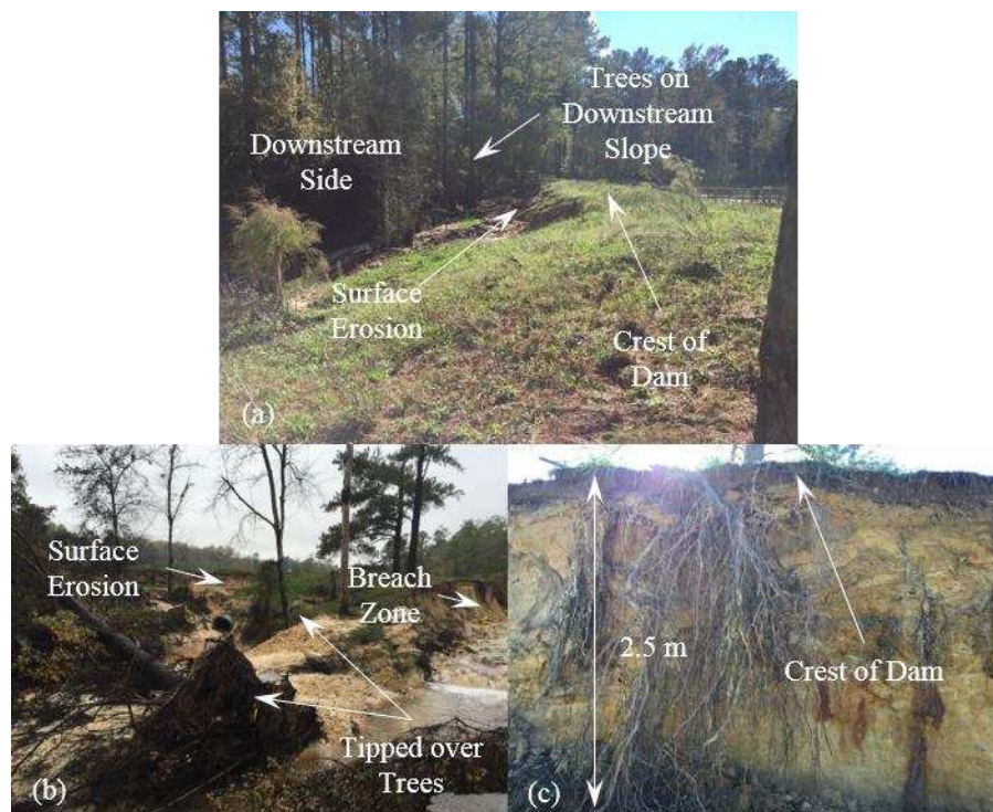
Figure 15. Vegetation on Dam B: (a) low grasses and small bushes on the dam crest, trees on downstream side slope (south view from crest), (b) tipped over trees near breach and zone of surface erosion (west view from downstream), and (c) presence of roots throughout the dam on the south breach wall (south view from breach).
