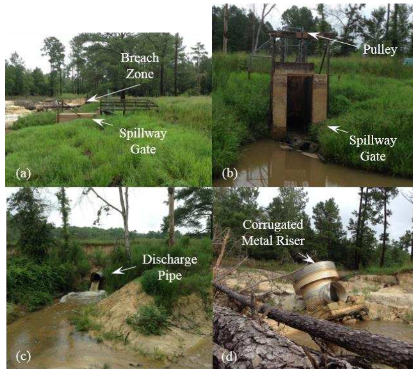
Figure 14. Spillway structures in Dam B: (a) location (view along the crest looking north), (b) concrete spillway gate (east view from upstream), (c) discharge pipe downstream from gate (east view from downstream), and (d) failed riser (northwest view from breach).
