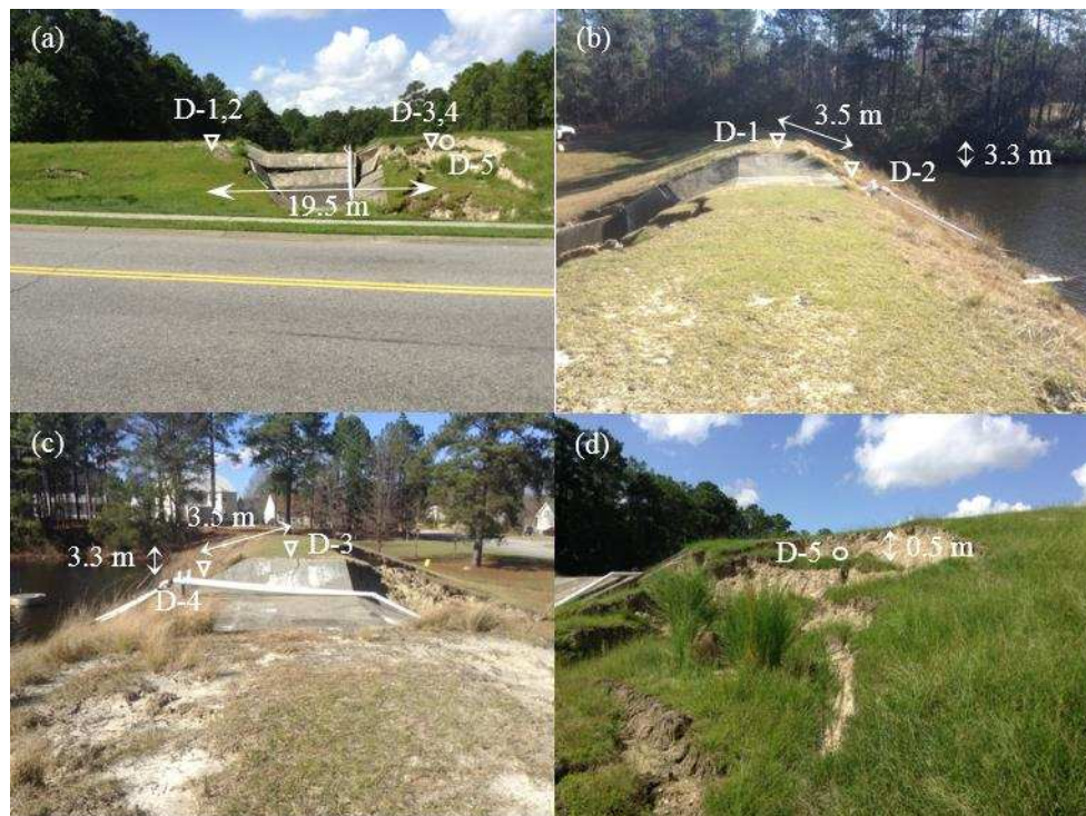
Figure 31. Sampling locations in Dam D: a) southwest view from Legion Drive, b) southeast view from the crest, c) northwest view from the crest, and d) southwest view from downstream side slope near the sliding zone (▽: vertical sample, ○: horizontal sample).
