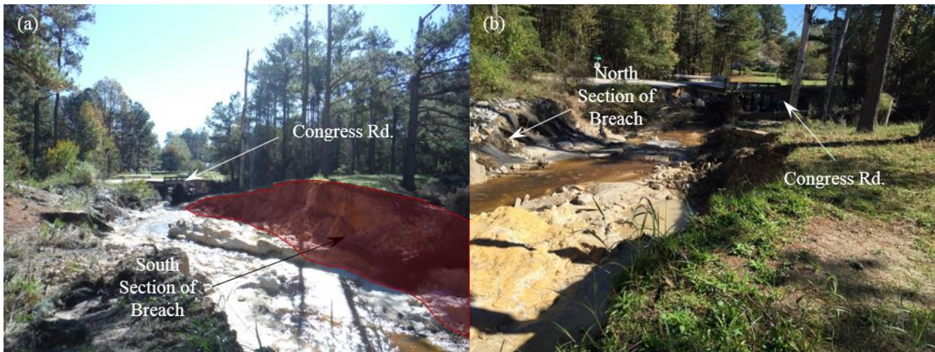
Figure 11. Breach section in Dam B: southeast views from (a) the north section of breach and (b) the south sections of the breach.
