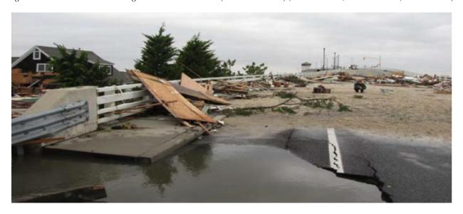
Figure 10. Foundation undermining at east abutment of Mantoloking Bridge (40.040058°N, 74.051886°W; GEER, 2014).
