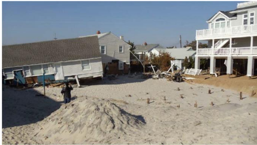
Figure 21. Timber piles remain in place after a home was sheared off in Pehola Park (39.610016N, 74.206657W, GEER, 2014).
