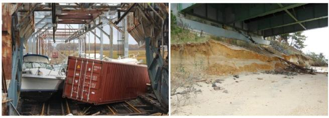
Figure 8. Morgan Drawbridge (left; NJ Transit) and Rt. 72 abutment erosion, looking south-east (right; NJDoT).
