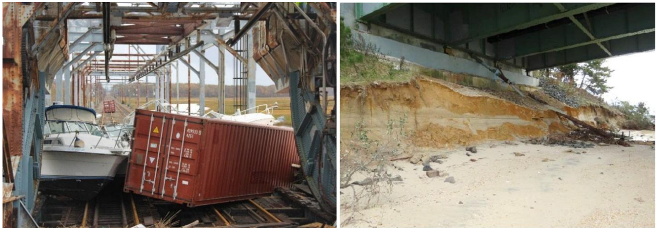
Figure 8. Morgan Drawbridge (left; NJ Transit) and Rt. 72 abutment erosion, looking south-east (right; NJDoT).
