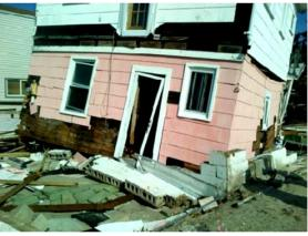
Figure 20. Undermining of beachfront retaining wall and loss of retained soil, Sea Gate, Brooklyn (left, 11/9/12); Destroyed CMU wall foundation, Breezy Point, Queens (right, 11/12/12). Photos by NYCDoB (GEER, 2014).
