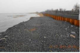
Figure 16. Earth embankment washouts in Queens, along Rockaway subway [A] line after Sandy with old LIRR infrastructure exposed (left) and post mitigation work (right). Photos by Khinda, ed. (2013).
