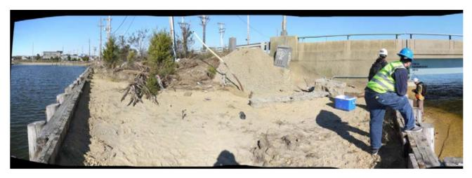
Figure 9. Erosion at Mathis Bridge southwest abutment (eastbound Rt37) (39.949350°N, 74.113902°W; GEER 2014).
