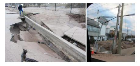
Figure 24. Scour undermining of street and utilities at Seaview Blvd, SI (40.579283°N, 74.077849°W, 11/4/12, GEER, 2014).
