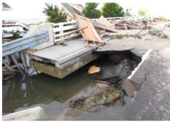
Figure 11. Mantoloking Bridge east abutment erosion (40.040058°N, 74.051886°W, Ocean Ct. Eng., 2012; GEER, 2014).
