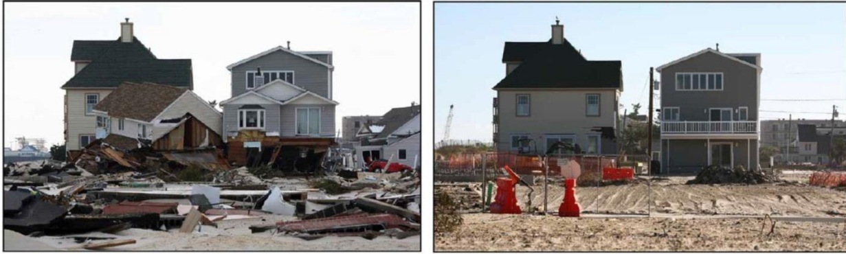
Figure 35. A home at Otely Beach, NJ, before (left) and after(right) rebuilding. Photos by NJ (2017).
