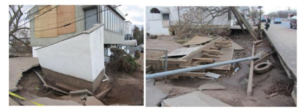
Figure 23. Scour undermining at Seaver Ave & Father Capodanno Blvd, SI (40.575944° N, 74.083015° W, 11/4/12). Damage to stair foundation and drain (left) and sidewalk, utilities, and light pole foundation (right). Photos by GEER (2014).
