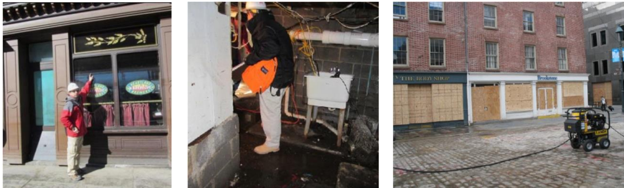
Figure 12. South Street Seaport (40.706685°N, 74.003554°W), 11/4/12: High water line on window of a restaurant (left); typical flooded basement (middle); flood damage (right). (GEER Report, 2014).
