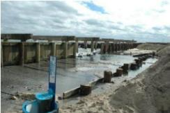
Figure 25. Bulkhead in Atlantic City, NJ: backfill soil washed away, exposing severely corroded tie rods (GEER, 2014).
