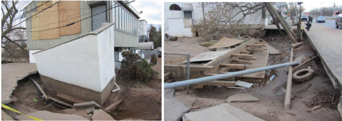
Figure 23. Scour undermining at Seaver Ave & Father Capodanno Blvd, SI (40.575944° N, 74.083015° W, 11/4/12). Damage to stair foundation and drain (left) and sidewalk, utilities, and light pole foundation (right). Photos by GEER (2014).
