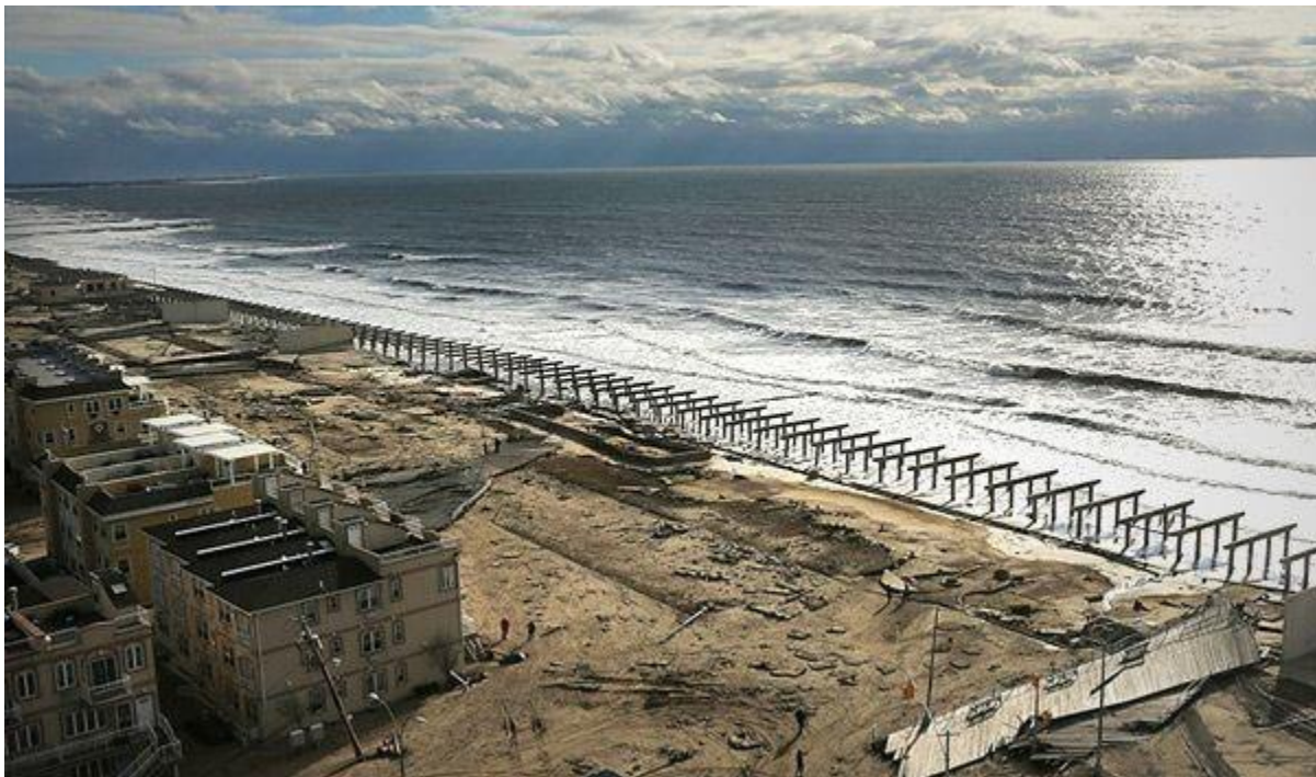
Figure 22. Damage to Boardwalk at Rockaway Beach, Queens (40.583445°N, 73.81553°W). Photo by cnbc.
