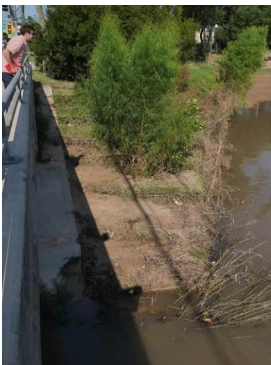
Figure 25. Buffalo Bayou evidence of scour a) Bridge abutment, and b) Downstream of Woodway Drive Bridge (September 9, 2017, 29.76457° N 95.45815° W).
