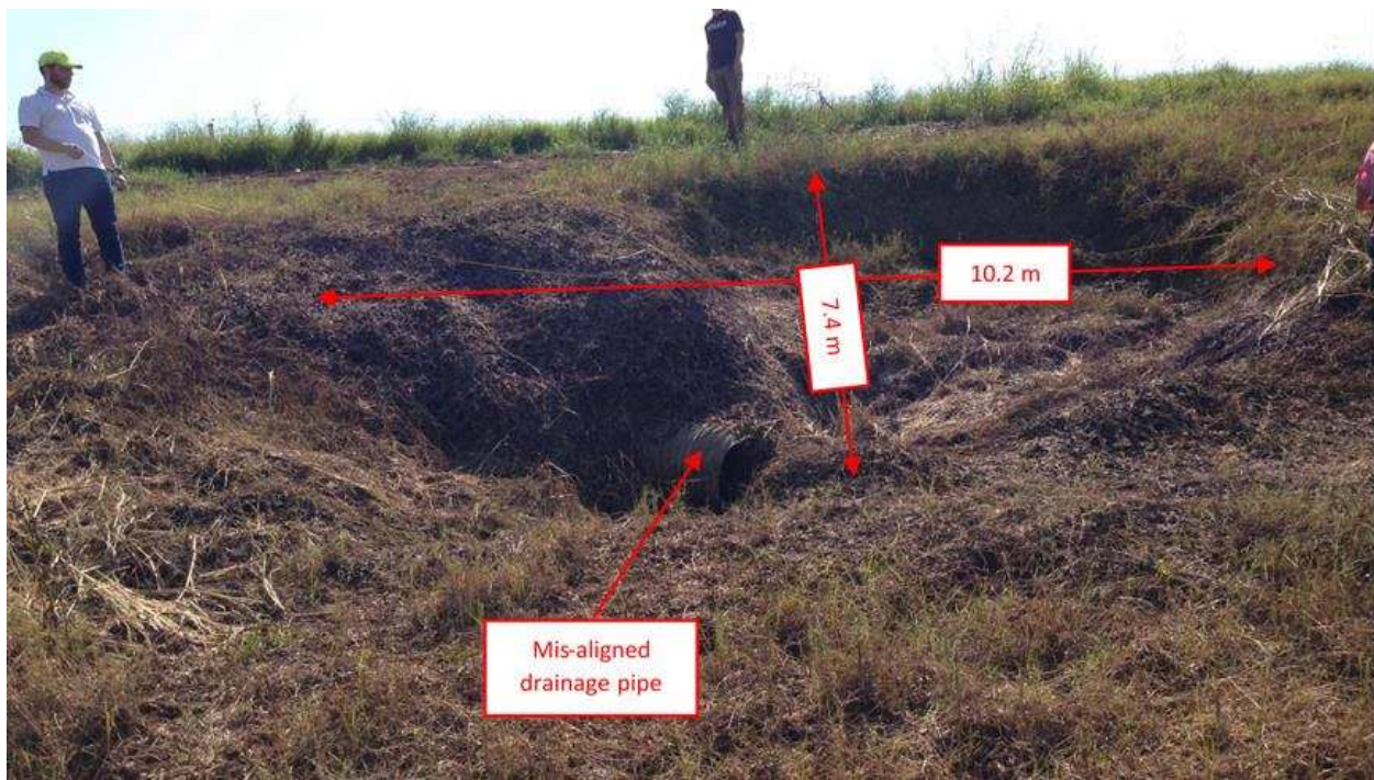
Figure 19. Sour hole at ruptured drainage pipe on Ditch H levee (September 10, 2017, 29.55759°N, 95.63768°W).
