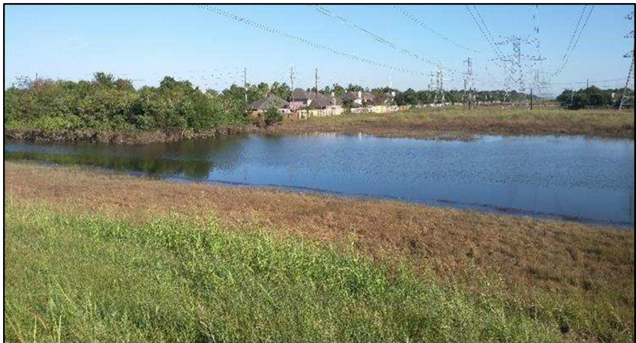
Figure 10. Flooded residential area in the southwest corner of the Barker Dam (September 9, 2017, 29.70706° N, 95.72835° W).
