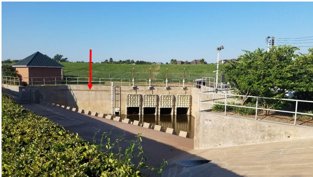
Figure 15. FCLID2 drainage outfall / pumping station basin, showing four 1.4 m (60 inch) flood gates, high water line at ~19.8 m (65 ft) gauge height, levee in background (September 10, 2017, 29.55509° N, 95.61779° W).
