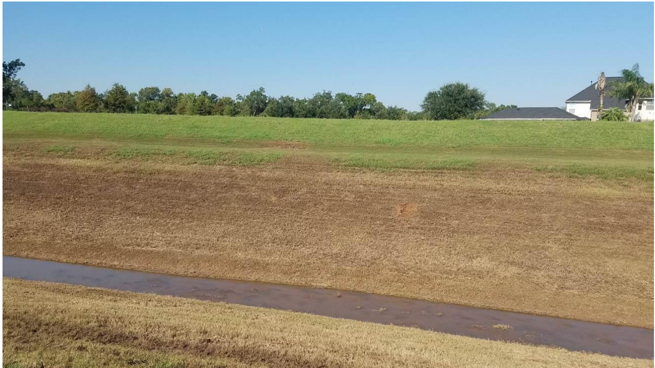
Figure 16. FCLID2 drainage ditch to Brazos River facing FBLID14 levee. High water line and persistent water lines visible on FBLID14 levee (September 10, 2017, 29.55292° N, 95.61820° W).
