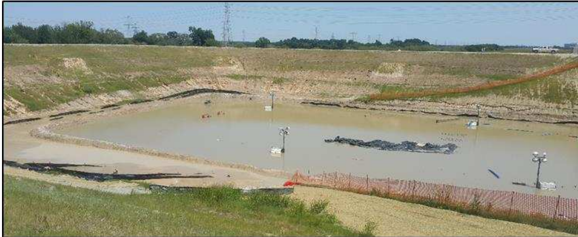
Figure 7. Interior of Addicks construction cofferdam for new outlet structure, flooded from Buffalo Bayou backwater; note erosion channels on slopes (September 9, 2017, 29.79063° N, 95.62586° W).
