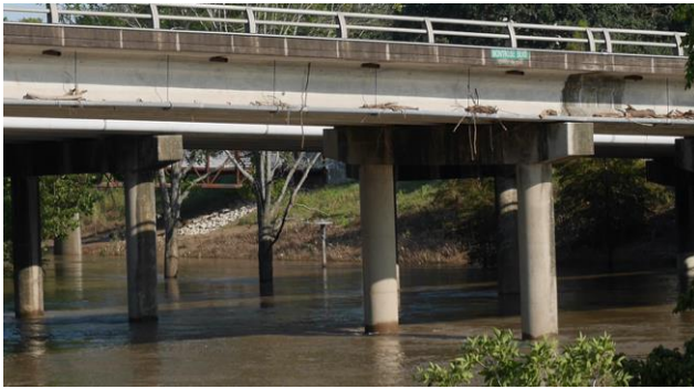
Figure 24. Buffalo Bayou evidence of bridge overtopping (flood debris:) a) Montrose Bridge (September 9, 2017, 29.76307° N 95.39377° W), and b) Memorial Bridge (September 9, 2017, 29.76219° N 95.38425° W).
