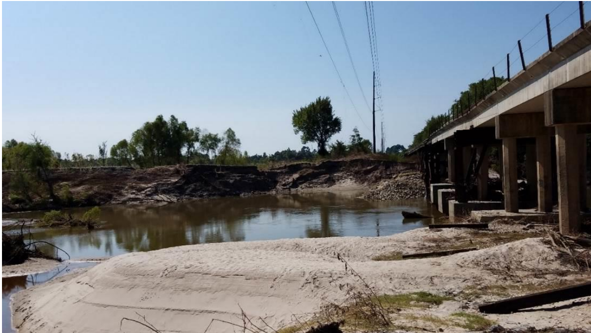
Figure 41. Bank erosion on the San Jacinto River downstream of I-45 and a railroad bridge parallel to the highway (September 11, 2017, Time 11:05 CDT, 30.24688° N, 95.45796° W).
