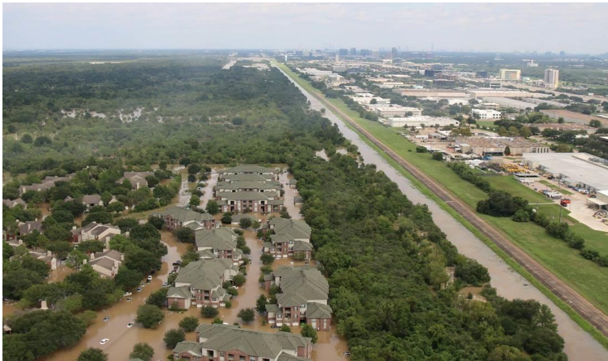
Figure 9. Aerial photograph of flooding within the Addicks Reservoir along the south auxiliary spillway (September 3, 2017, 29.79222° N, 95.68830° W, USACE photograph).
