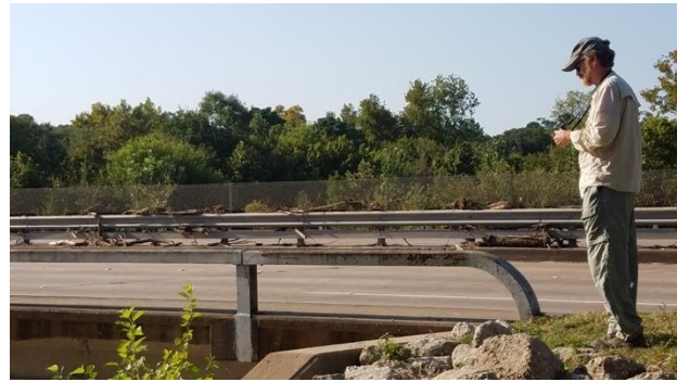
Figure 24. Buffalo Bayou evidence of bridge overtopping (flood debris:) a) Montrose Bridge (September 9, 2017, 29.76307° N 95.39377° W), and b) Memorial Bridge (September 9, 2017, 29.76219° N 95.38425° W).
