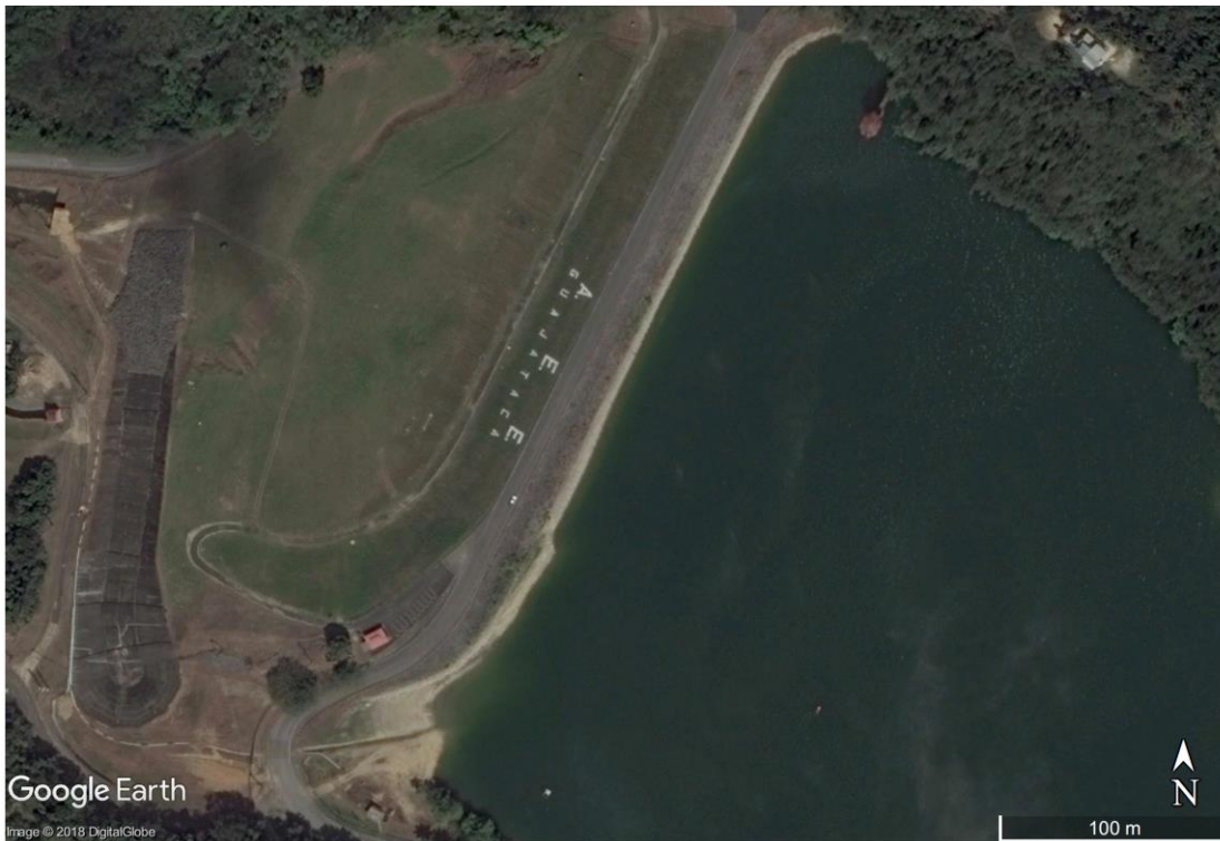
(a) Aerial photograph of dam before Hurricane Maria (March 2017, Source: Google Earth).
