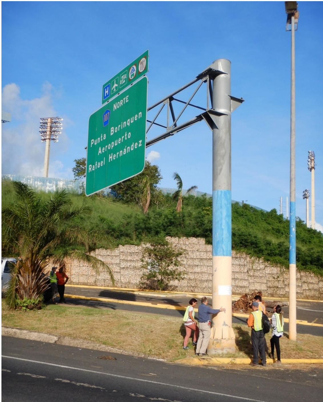
Figure 24. Photo of cantilevered sign foundation failure (GEER Mission Site F2; Silva-Tulla et al. 2018).
