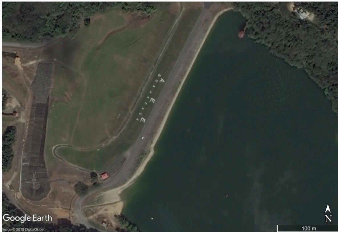
(a) Aerial photograph of dam before Hurricane Maria (March 2017, Source: Google Earth).
