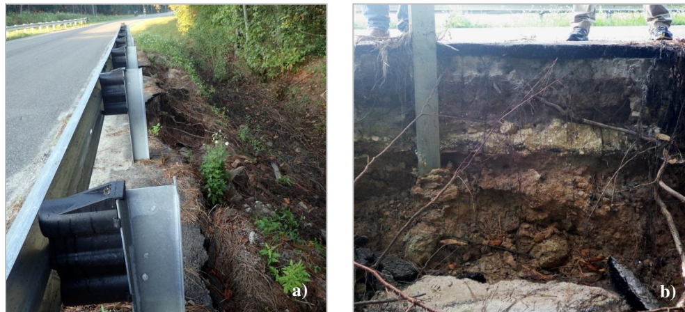
Figure 17: Erosion damage of the northern section of Lake Hampton Road at the Pigeon River crossing north of the dam near 30°46'45.19"N latitude and 81°58'24.6"W longitude.
