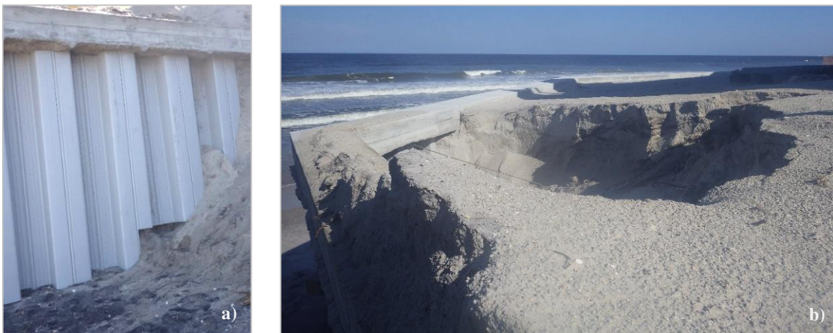
Figure 12: Sheet pile retaining wall failure from undercutting at 29°56'58.16"N latitude 81°18'11.96"W longitude, showing: (a) the exposed wall base, and (b) a funnel-shaped depression following basal soil escape (Hudyma et al., 2017).
