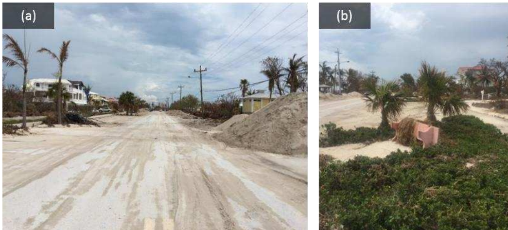
Figure 12. (a) Large volumes of sediment were deposited on Sombrero Beach Road (facing east) and (b) a concrete bench was overturned, trapping debris on its side (collected September 26, 2017; location 24^{\circ}41'33.01''\text{N} , 81^{\circ}5'5.57''\text{W} ).
