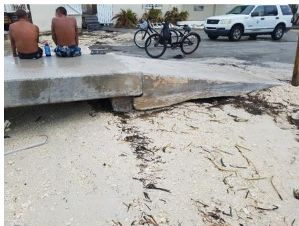
Figure 11. A concrete structure located on the eastern edge of Simonton Beach was undermined due to scour around the structure (collected September 27, 2017; location 24^{\circ}33'43.32''\text{N} , 81^{\circ}48'20.22''\text{W} ).
