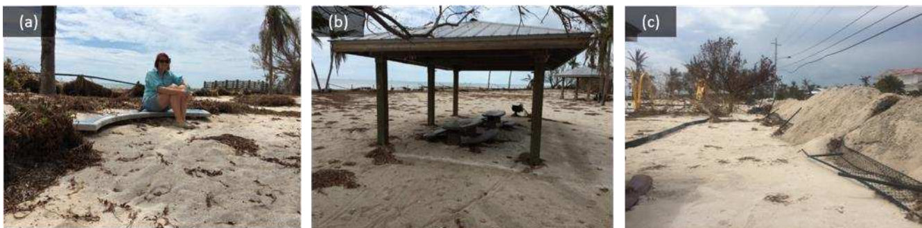
Figure 16. (a) Concrete park benches were nearly buried with sand (approximately 2 m), (b) some park structures were only mildly damaged and buried with sediment, (c) while others were severely damaged and in need of repair (collected September 26, 2017; location 24^{\circ}41'32.20''\text{N} , 81^{\circ}5'4.09''\text{W} ).
