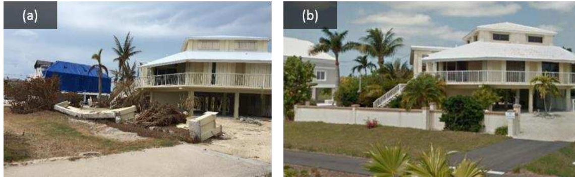
Figure 14. (a) A wall located in front of a home on Sombrero Beach Road collapsed during Hurricane Irma (collected September 26, 2017; location 24^{\circ}41'34.26''N , 81^{\circ}5'0.93''W ); (b) the pre-existing structure appeared to be intact prior to the storm. Map Data: Google (2018).
