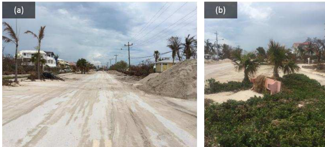
Figure 12. (a) Large volumes of sediment were deposited on Sombrero Beach Road (facing east) and (b) a concrete bench was overturned, trapping debris on its side (collected September 26, 2017; location 24°41'33.01"N, 81°5'5.57"W).
