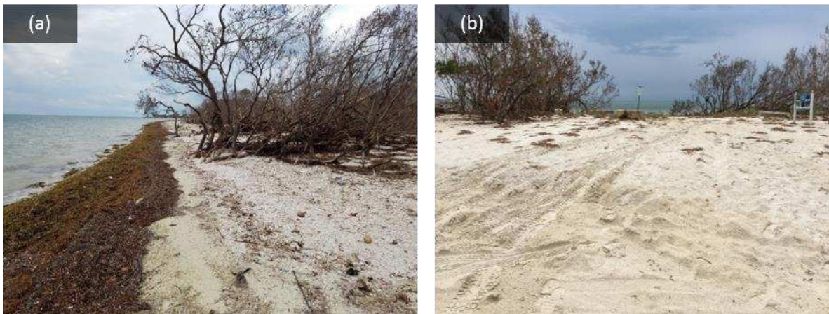
Figure 18. (a) The beach width was narrowed due to erosion and algae washed up on the beach, and (b) sediment approximately 0.3 m in depth was deposited in the beach access area (collected September 26, 2017; location 24^{\circ}43'48.42''N , 81^{\circ}0'5.81''W ).
