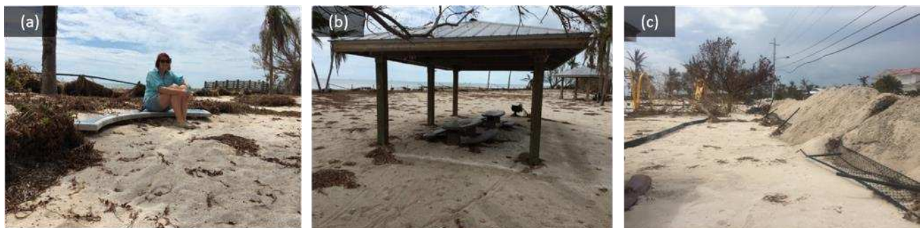
Figure 16. (a) Concrete park benches were nearly buried with sand (approximately 2 m), (b) some park structures were only mildly damaged and buried with sediment, (c) while others were severely damaged and in need of repair (collected September 26, 2017; location 24^{\circ}41'32.20''N , 81^{\circ}5'4.09''W ).
