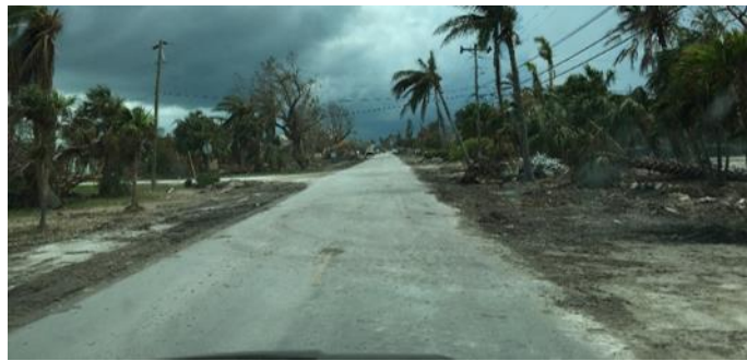
Figure 17. Sand and debris were deposited on Coco Plum Drive (collected September 26, 2017; location 24^{\circ}43'34.52''N , 81^{\circ}0'36.53''W ).
