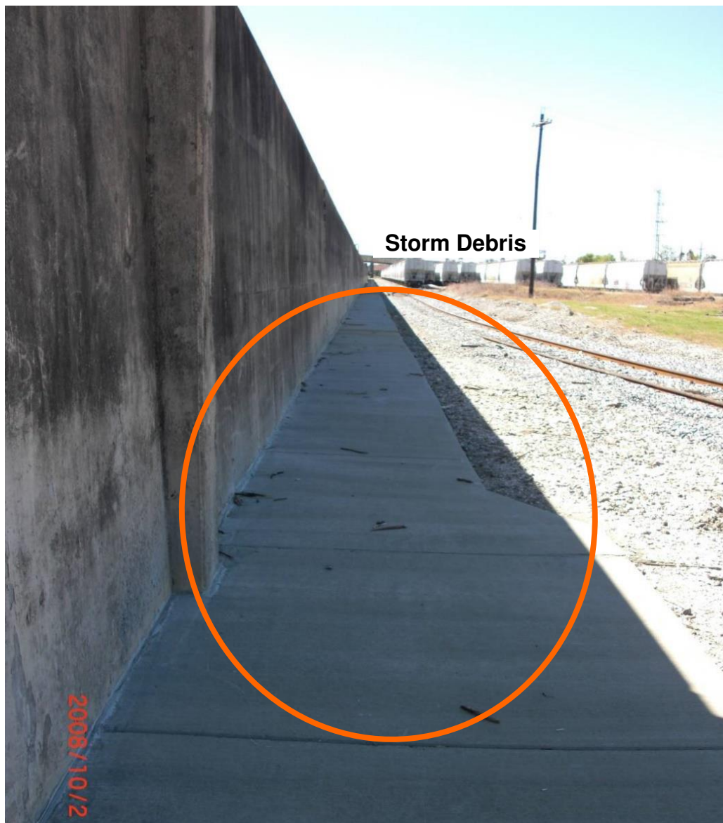
Figure 23. Photograph from October 2, 2008, of IHNC West T-wall (same section as shown during Gustav in Figures 20 and 21). (October 2, 2008, 29.970° N, 90.026° W)
