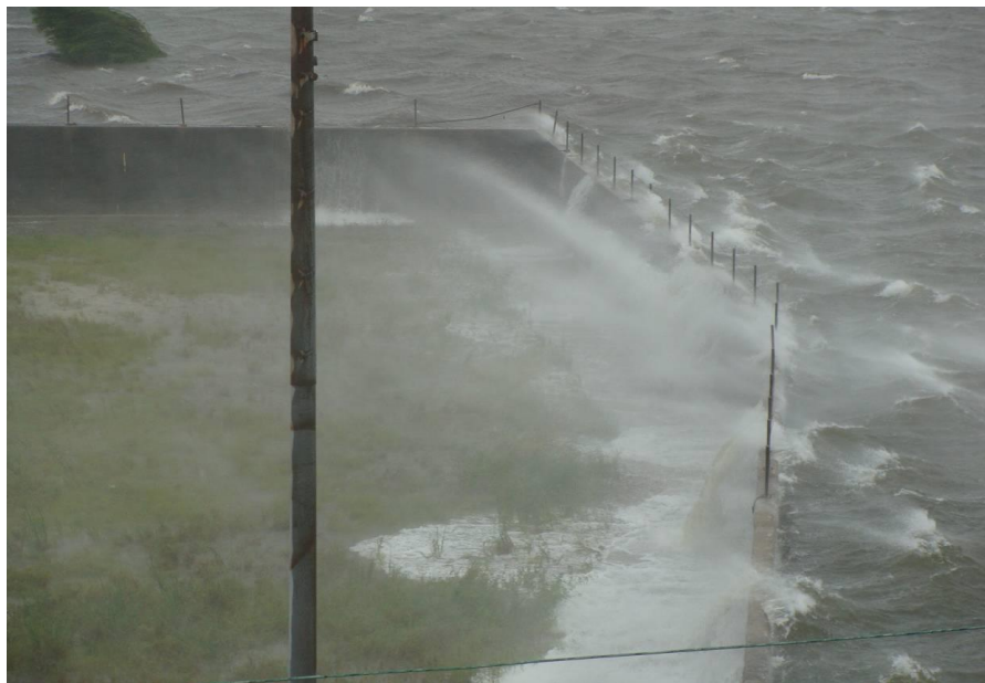
Figure 22. Gustav's storm surge along IHNC East, taken from Claiborne Ave. Bridge looking north at T-wall southeast on September 1, 2008. (September 1, 2008, 29.969° N, 90.027° W, USACE)
