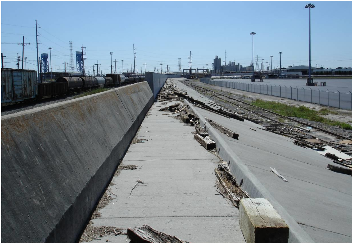
Figure 6. I-wall and splash apron, IHNC west along France Road; new L-wall and splash apron in background. (October 2, 2008, 90.0272° W, 90.0272° W)
