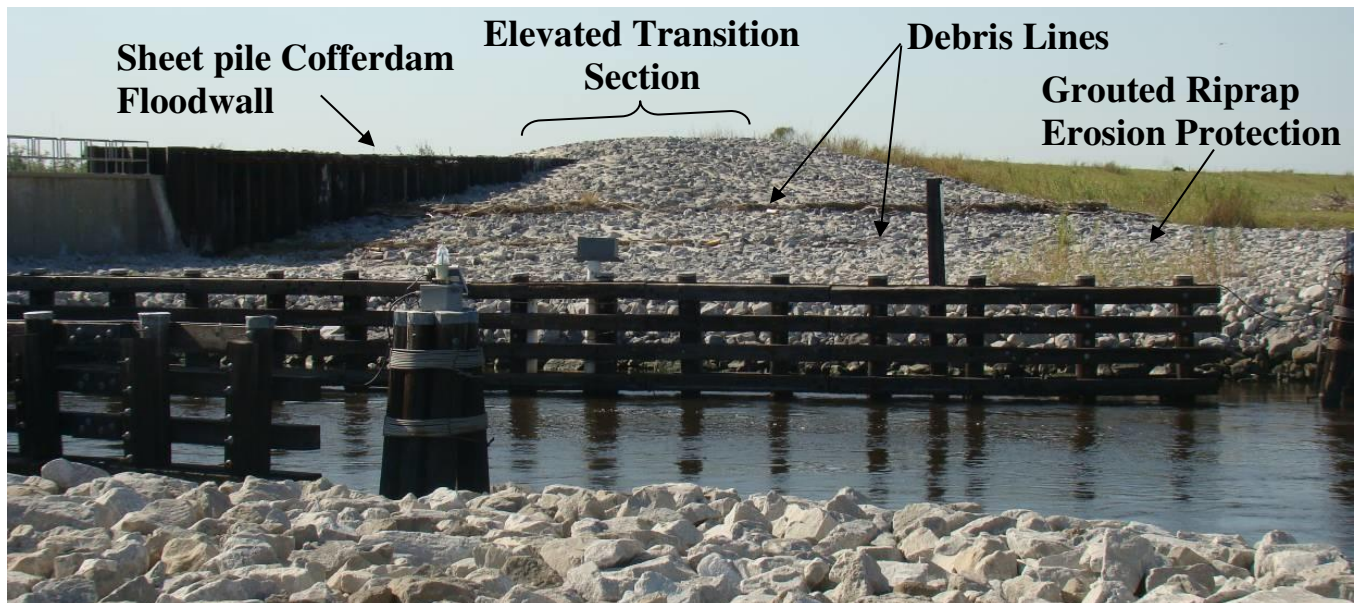
Figure 14. Bayou Dupree gate, northwest flank, MRGO side, looking east. The lower debris line may represent the high-water level during Hurricane Ike. (October 2, 2008, 29.9352° N, 89.8358° W)
