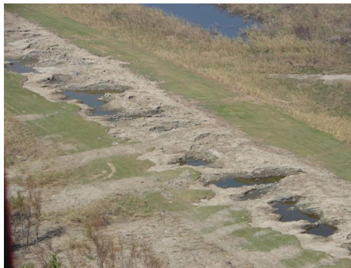
Figure 11. Post-Katrina MRGO frontage levee. (October 14, 2005, ~89.8° W, ~29.9° N, L. Harder)
