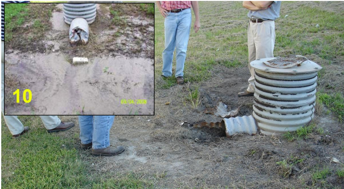
Figure 29. Relief well cover, as of October 2008, with inset taken from the USACE Hurricane Gustav Damage Assessment Team SITREP on September 5, 2008. (October 2, 2008, 30.0249° N, 90.0294° W)
