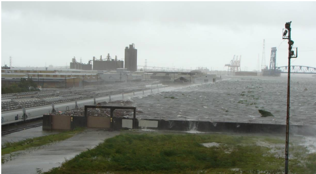
Figure 21. Photograph from September 1, 2008, of Gustav's storm surge. Photograph taken from Claiborne Ave. Bridge looking north. The waves are overtopping the T-wall. (September 1, 2008, 29.969° N, 90.027° W, USACE)
