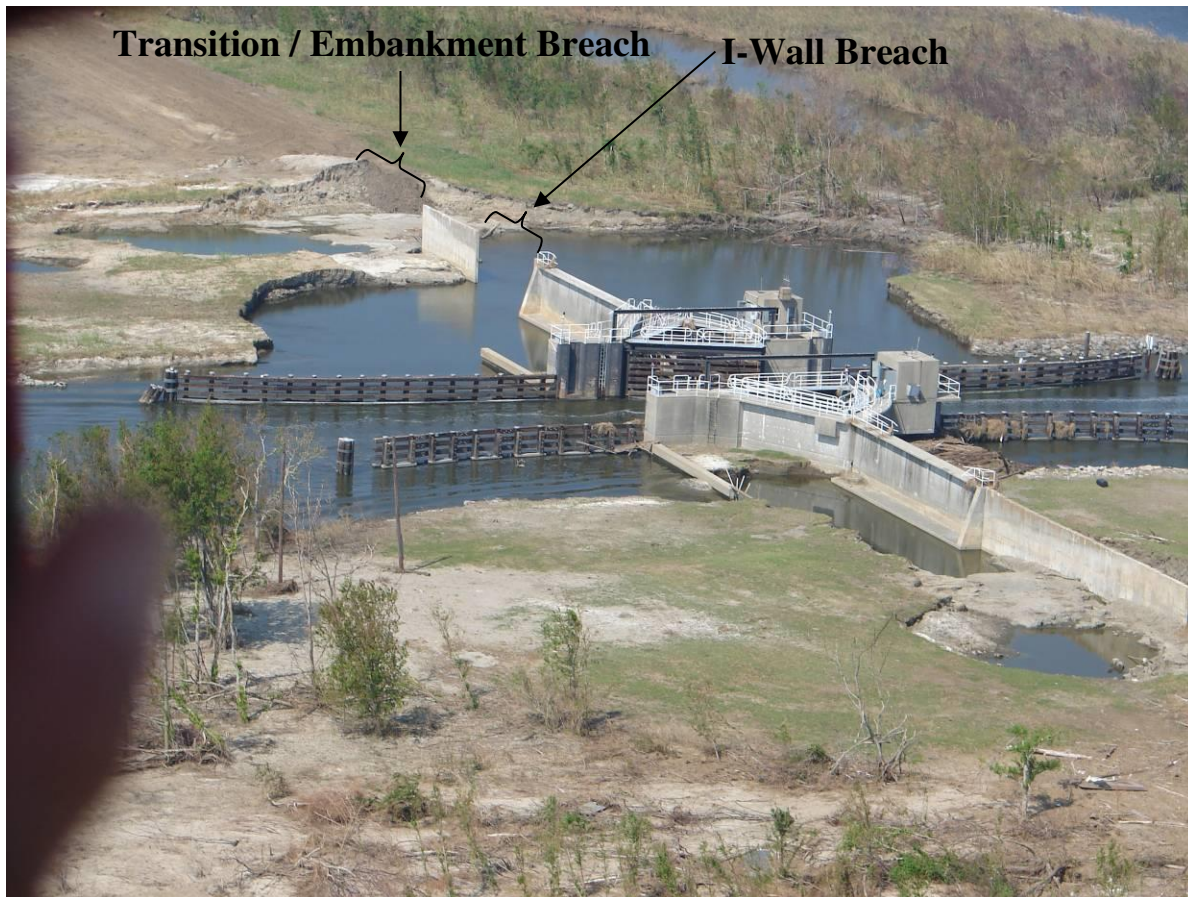
Figure 13. Post-Katrina Bayou Dupree gate. (October 14, 2005, 29.935° N, 89.837° W, L. Harder)
