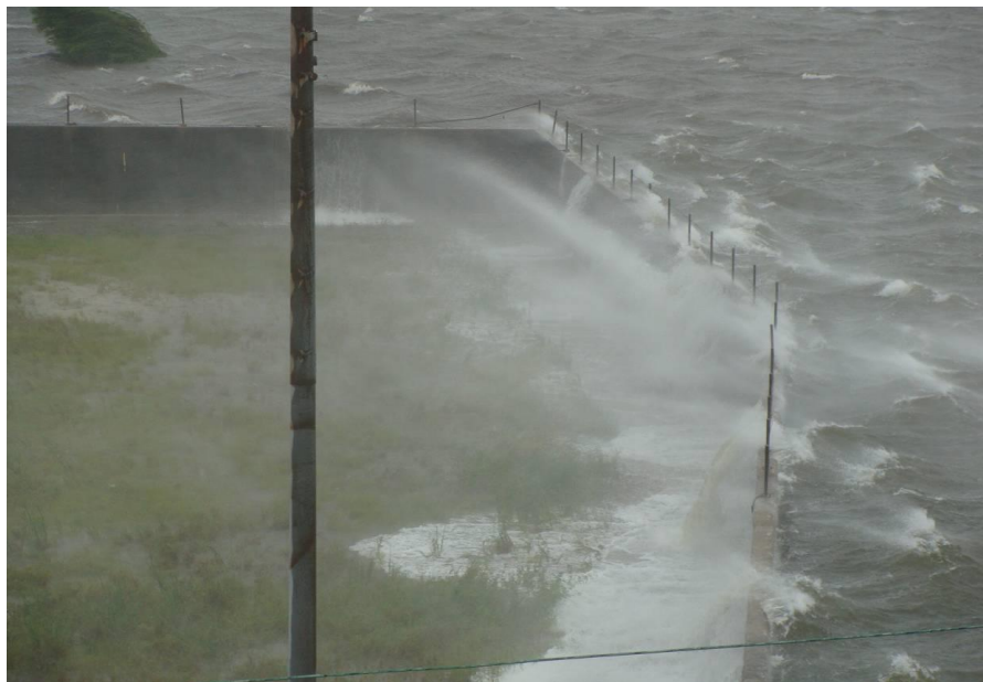
Figure 22. Gustav's storm surge along IHNC East, taken from Claiborne Ave. Bridge looking north at T-wall southeast on September 1, 2008. (September 1, 2008, 29.969° N, 90.027° W, USACE)
