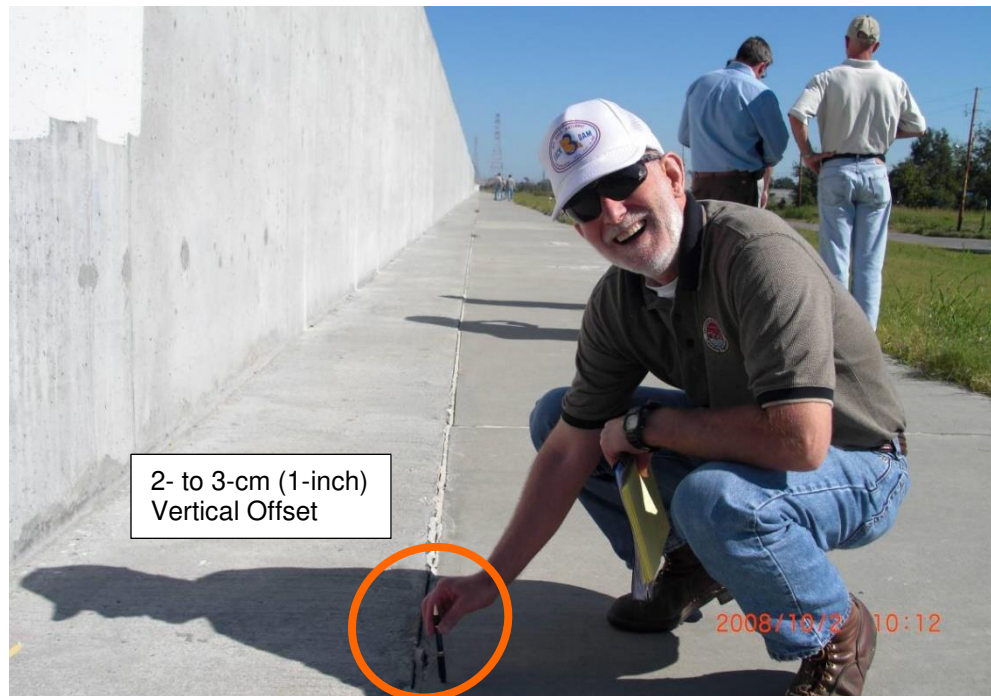
Figure 27. New T-wall section along the east side of the IHNC between Claiborne and Florida Avenues (shown in Figure 23 during Gustav). (October 2, 2008, 29.9691° N, 90.0236° W)
