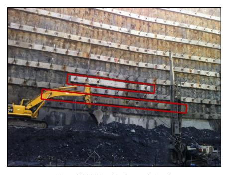
Figure 11. Additional Anchors on Section 3.
