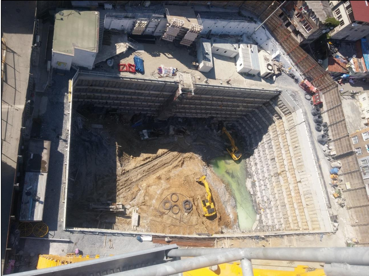
Figure 14. An Aerial View of the Project Site.
