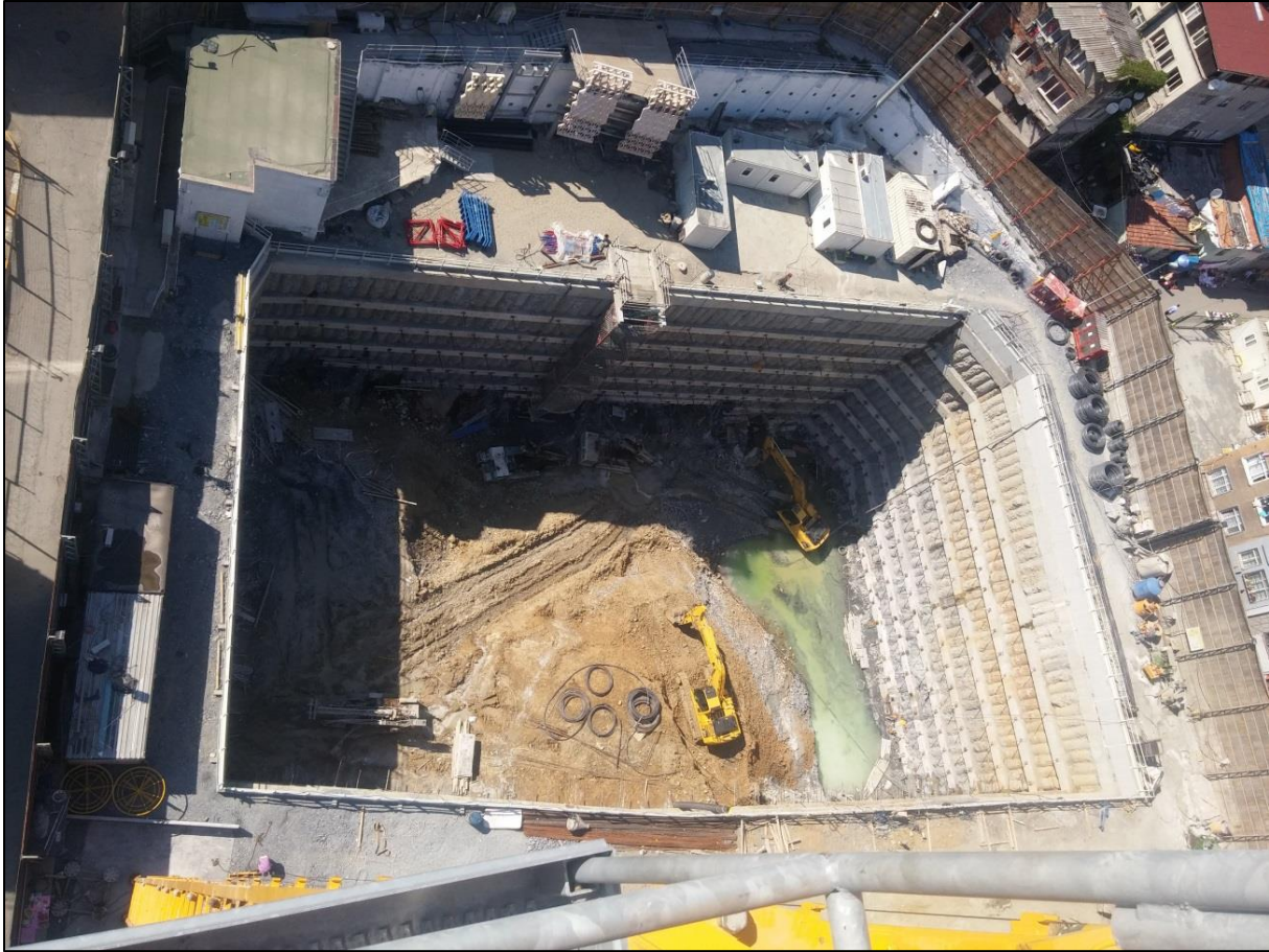
Figure 14. An Aerial View of the Project Site.
