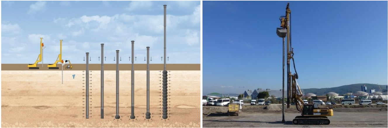
Figure 8. Construction methodology of RAP Impact elements and a view from the field construction.
