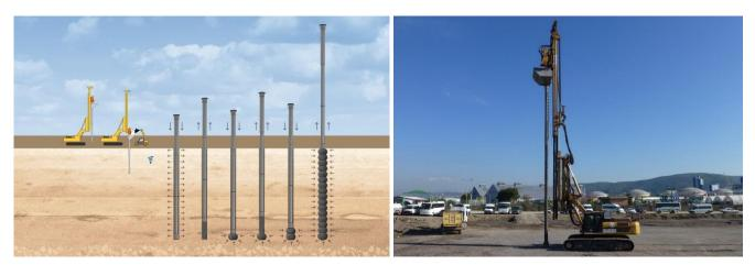
Figure 8. Construction methodology of RAP Impact elements and a view from the field construction.
