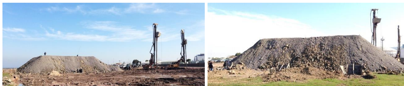
Figure 15. The test embankment field photos.
