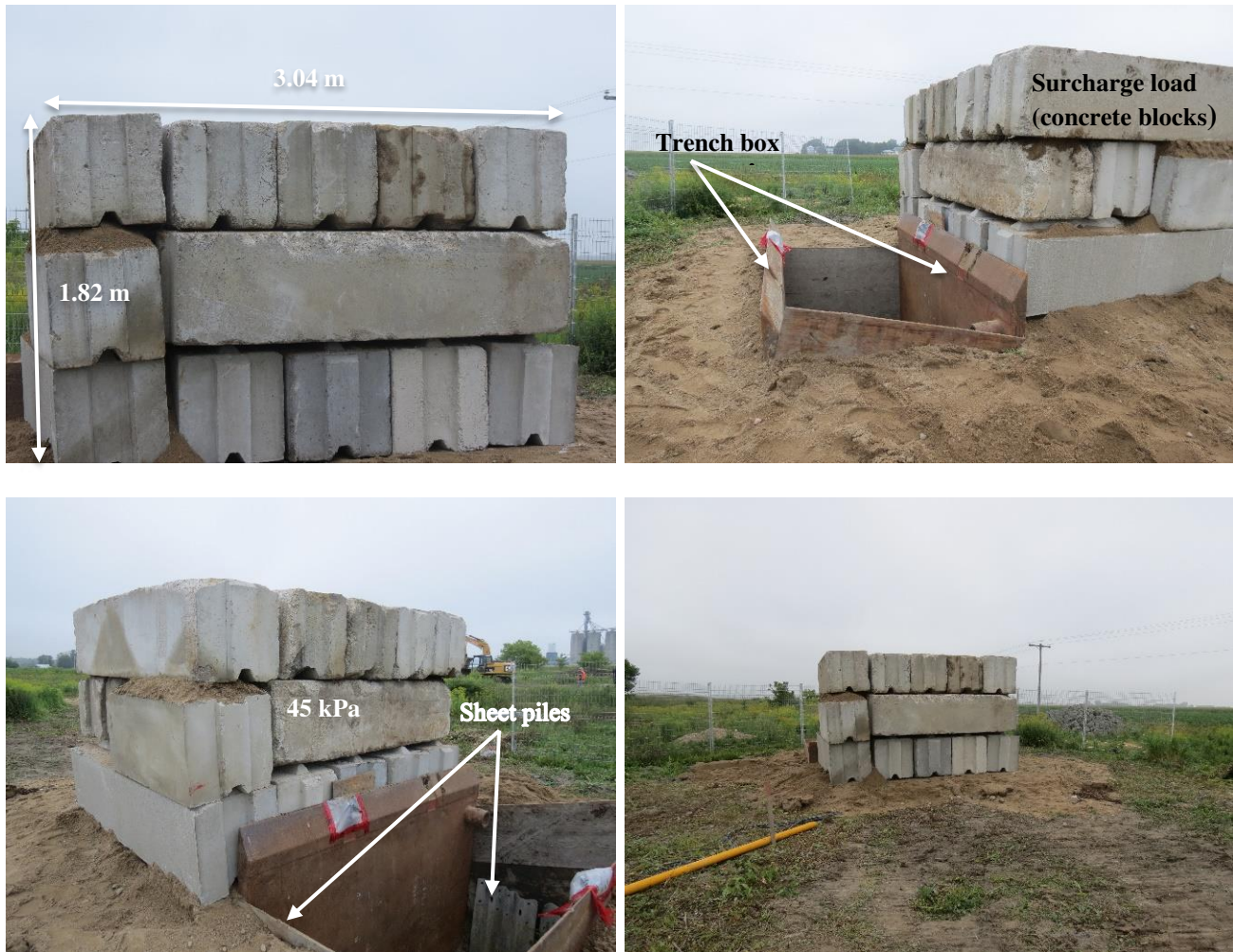
Figure 14. Concrete blocks (surcharge load) installed on one side of the trench.
