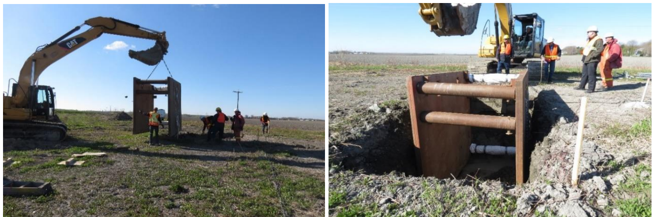
Figure 10. Installation of the first (lower) trench box into the trench.
