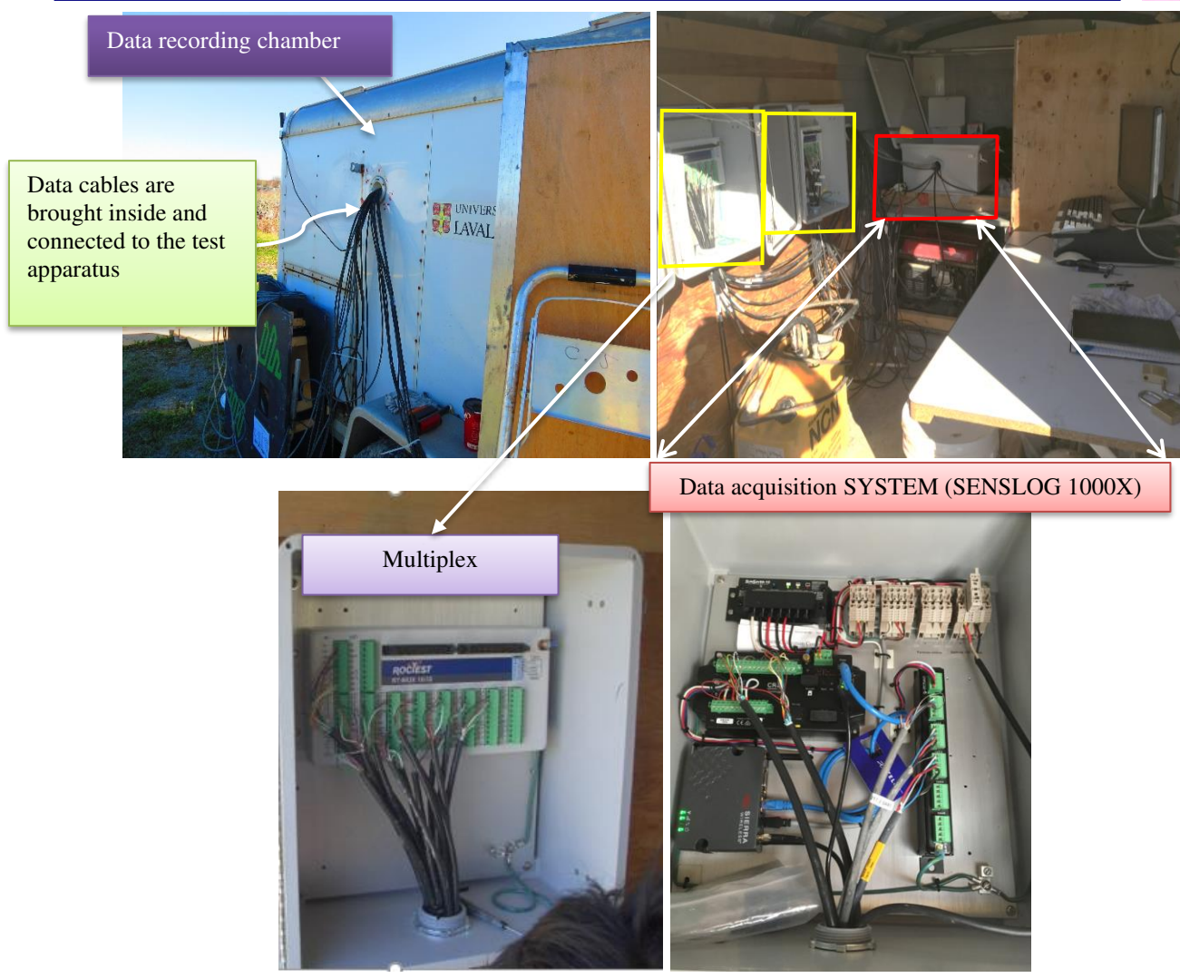
Figure 15. Components of the data recording unit at the experimental site.
