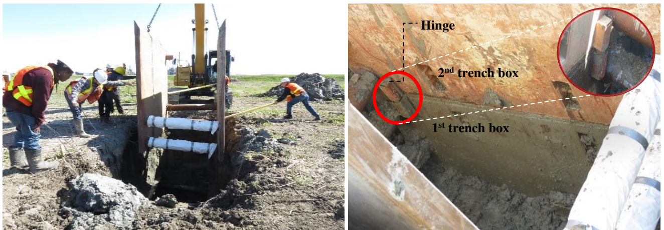
Figure 12. Second (upper) trench box is being placed on top of the first (lower) box in the trench.
