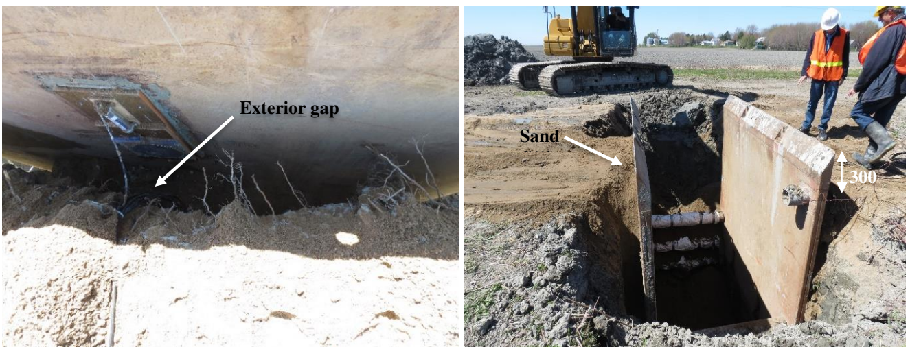
Figure 13. Sand was used to fill the space between the shoring exterior wall and the surrounding soil.
