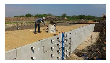
Figure 30. Construction of the MSE wall.
