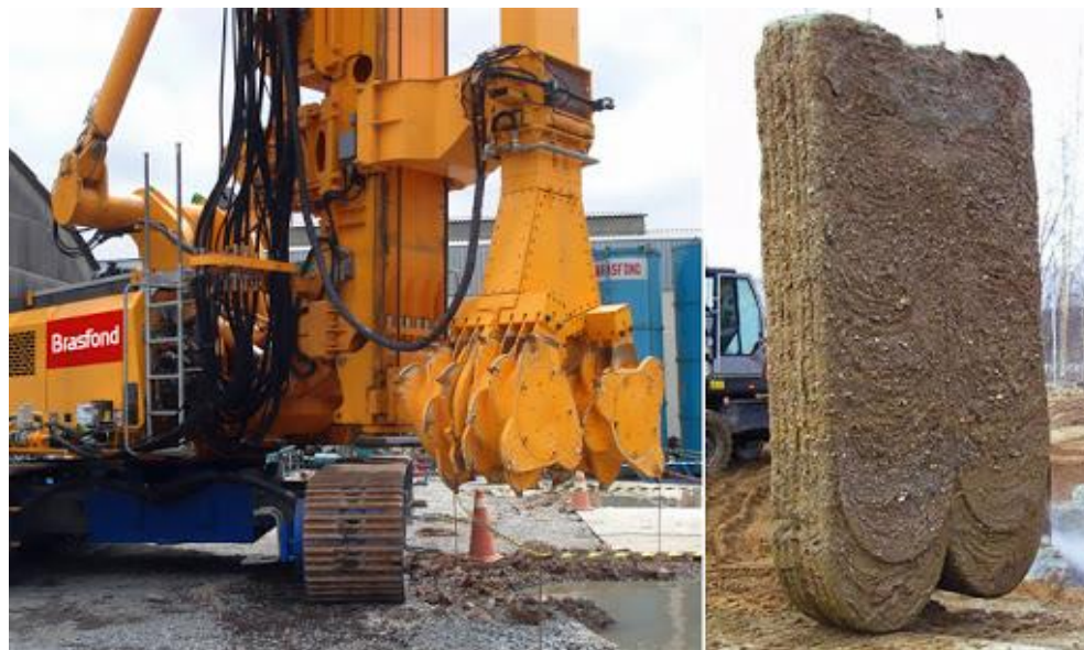
Figure 1. Cutter soil mix (CSM) rig and CSM panel.
