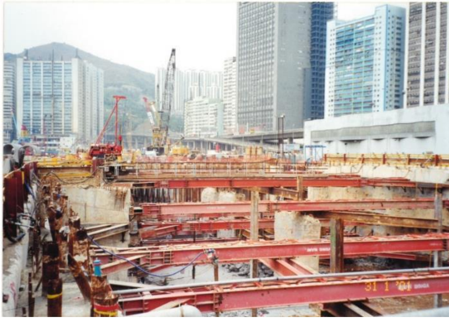
Figure 5. Excavation works taken place for Tsuen Wan West Station in 2001.
